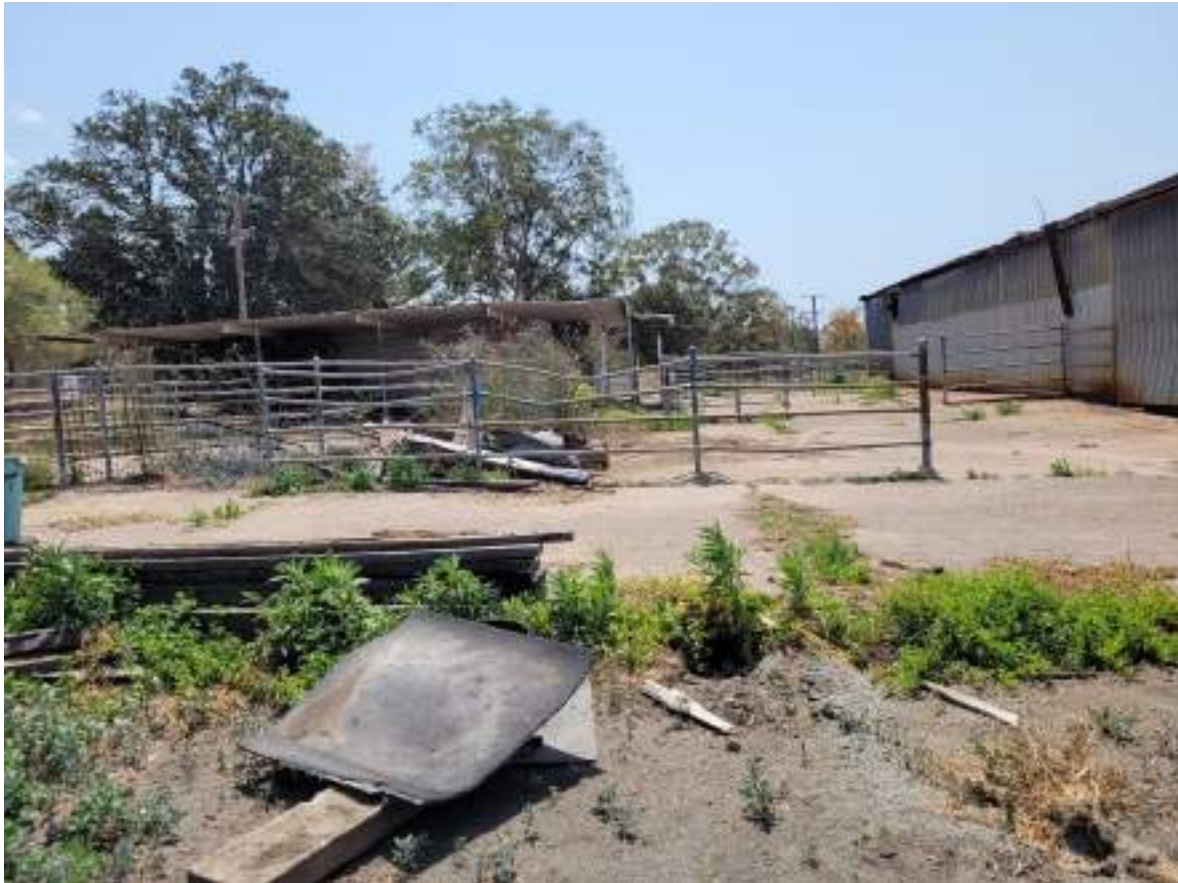
Plate 2-4. Livestock fencing and general rubbish that would need to be removed. View from the south.
