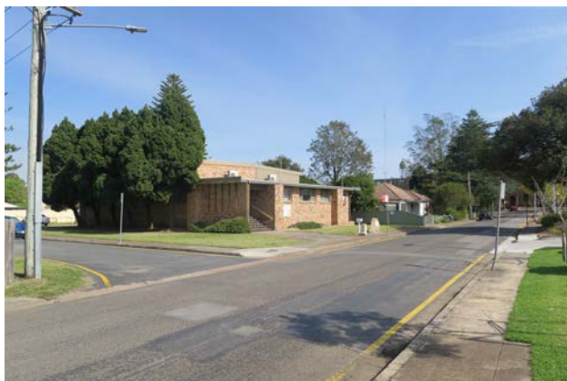
Figure 21: View along Grant Street from Old Rose Street corner. The proposed development adopts the same setback as both the Polish Club and the existing residence.
