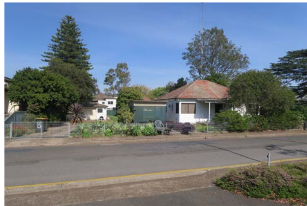
Figure 20: View of the existing building from the north of Grant Street.
