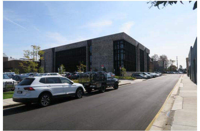
Figure 13: South east view of Maitland Council building from Devonshire Street; the archetypal form intended for this section of Central Maitland.
