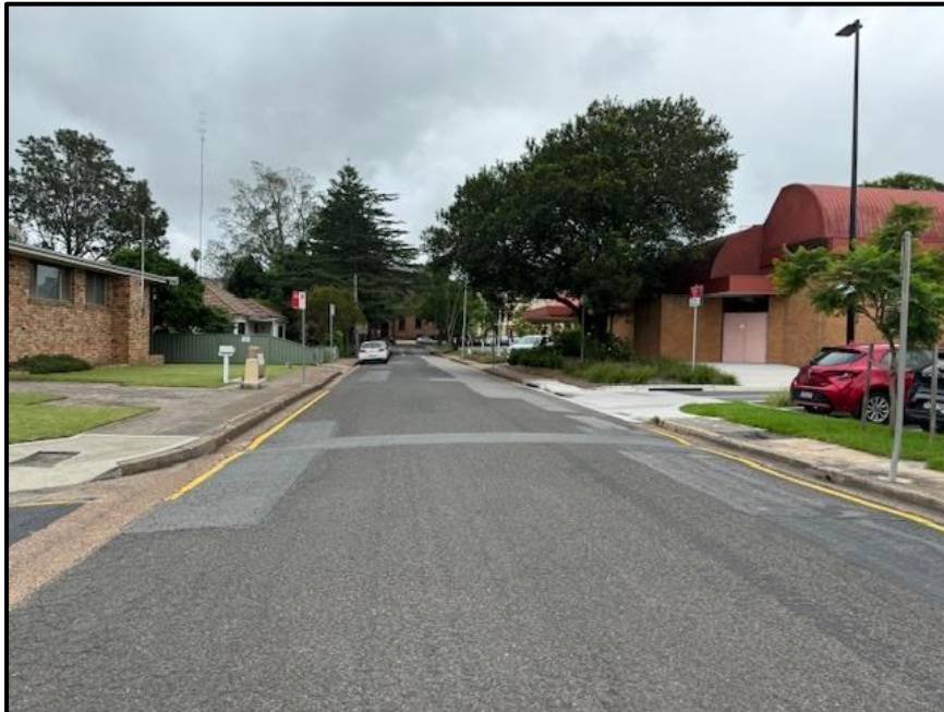
Photo 1 – View looking west on Grant Street showing typical cross section.
