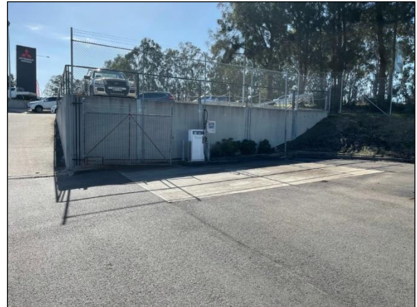
Figure 25: Bowser and UST location, looking north-east.
