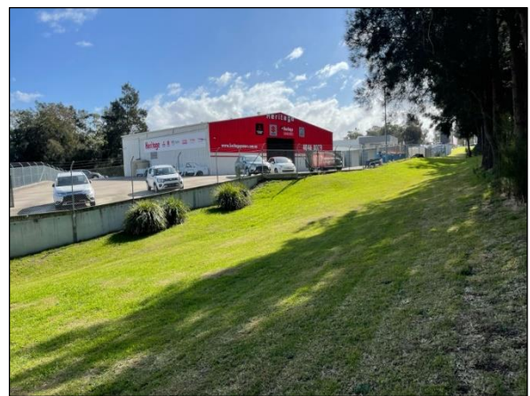
Figure 27: Detailing workshop in the southern portion of the site, looking north-west.
