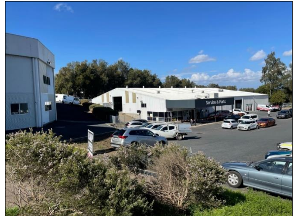
Figure 13: Warehouse in the central portion of the site, looking south-east.
