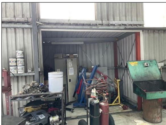
Figure 22: Former flammable liquids storage, northern side of warehouse
