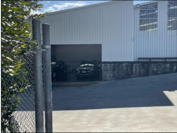
Figure 24: Wash bay attached to warehouse, looking north.
