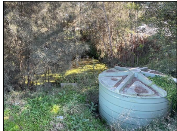
Figure 31: Water storage tank adjacent to the sediment dam (background), south of main developed area, looking west. Receives surface water runoff from main site (rainwater etc). Discharge from dam to surface water body
