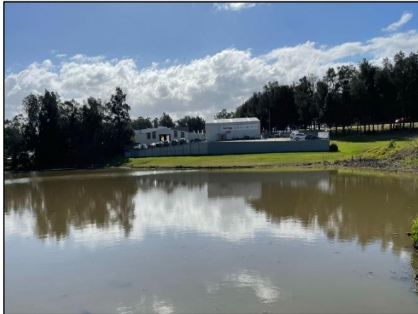
Figure 30: Above grade fill platform in the southern portion of the site, looking north.
