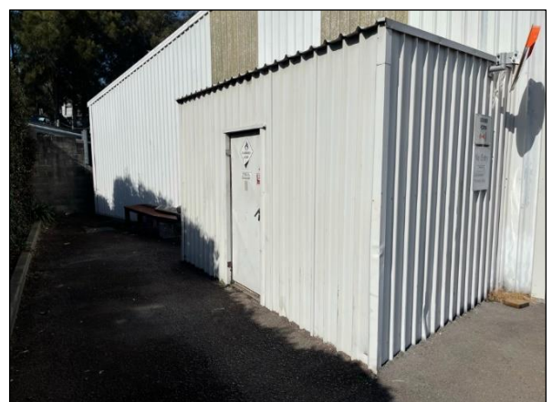
Figure 21: Former flammable liquids storage, northern side of warehouse
