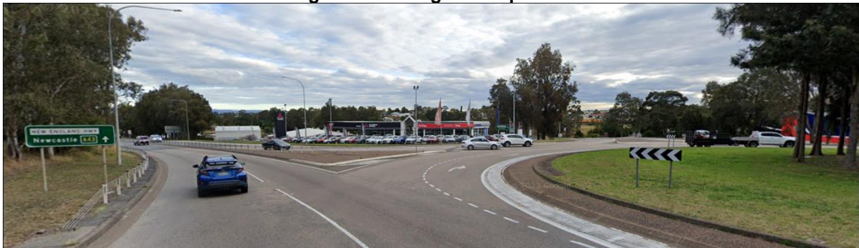
Figure 5 Existing Site Exposure
