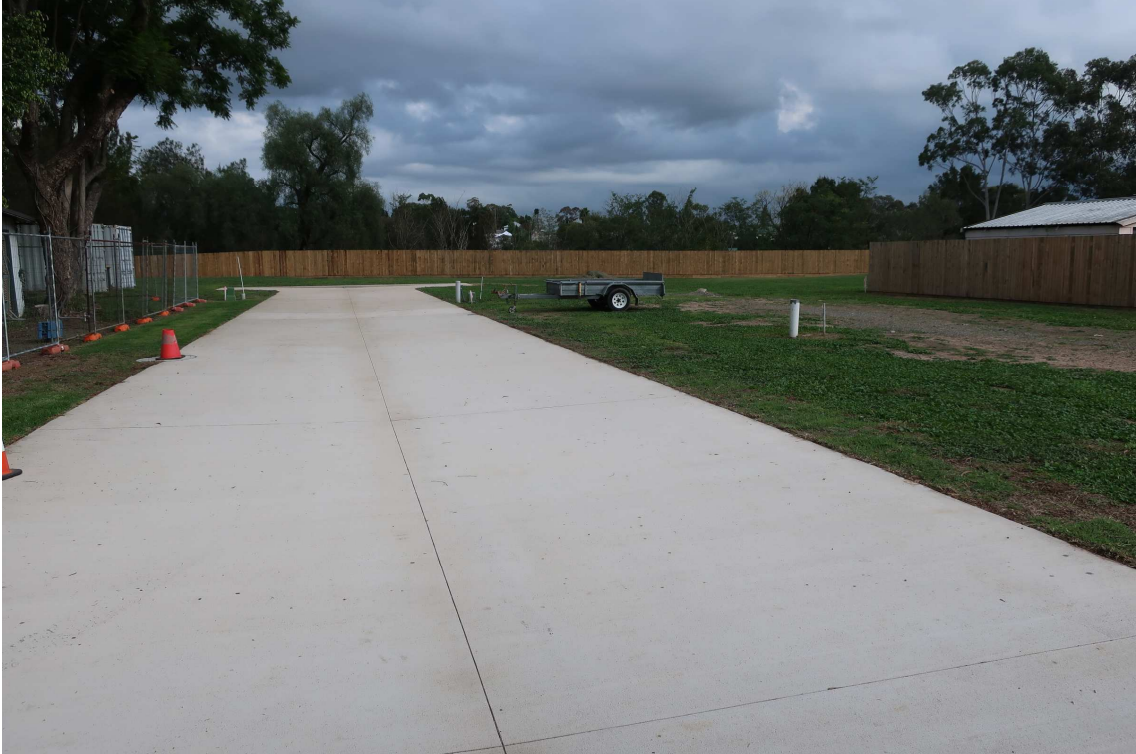
Figure 8: View of driveway right of carriage way to the west
