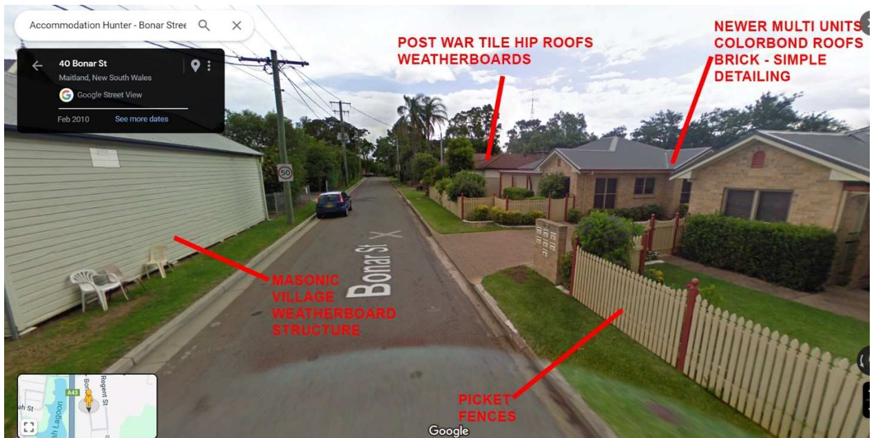
Figure 16 - View of Bonar Street Looking South. 44 Bonar Street to the right is multi dwelling development. Simple heritage detailing, hip and gable roofs with colorbond. Picket fences are used to formalize the front yards. Double hung windows present to the front facades. Gable ends prominent in front façade.
