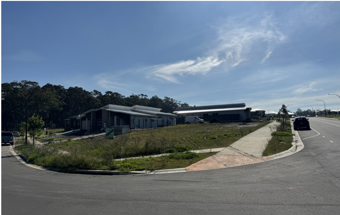
PHOTO 1 - SITE PHOTO LOOKING NORTHWEST
