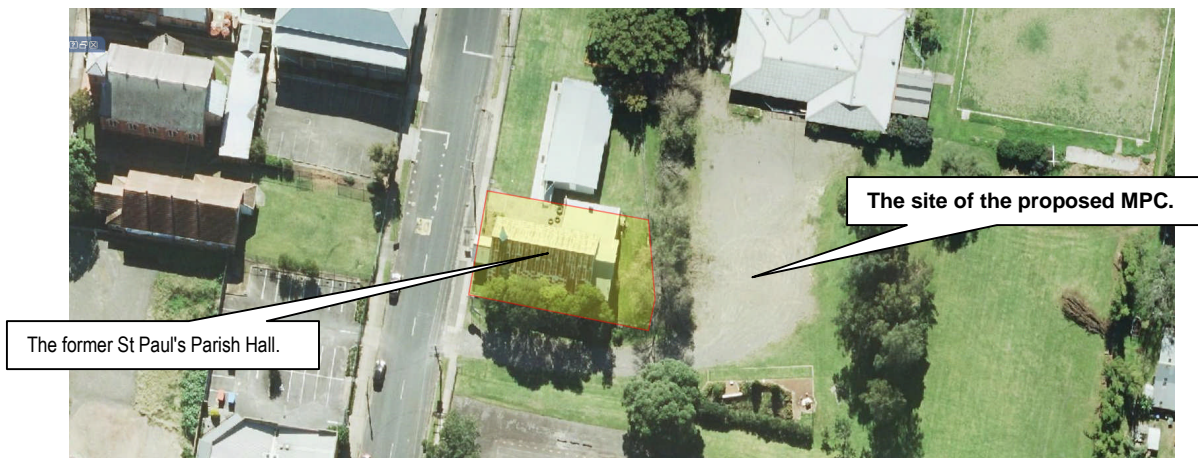
Plate 1: Aerial view of the site and neighbouring buildings. (Six Maps accessed 11/05/21)
