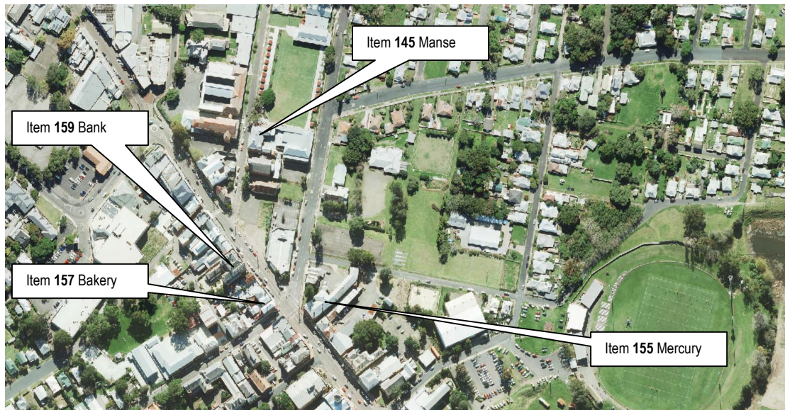
Plate 19: The Maitland City Centre showing the subject site & nearby heritage items. (Six Maps)
