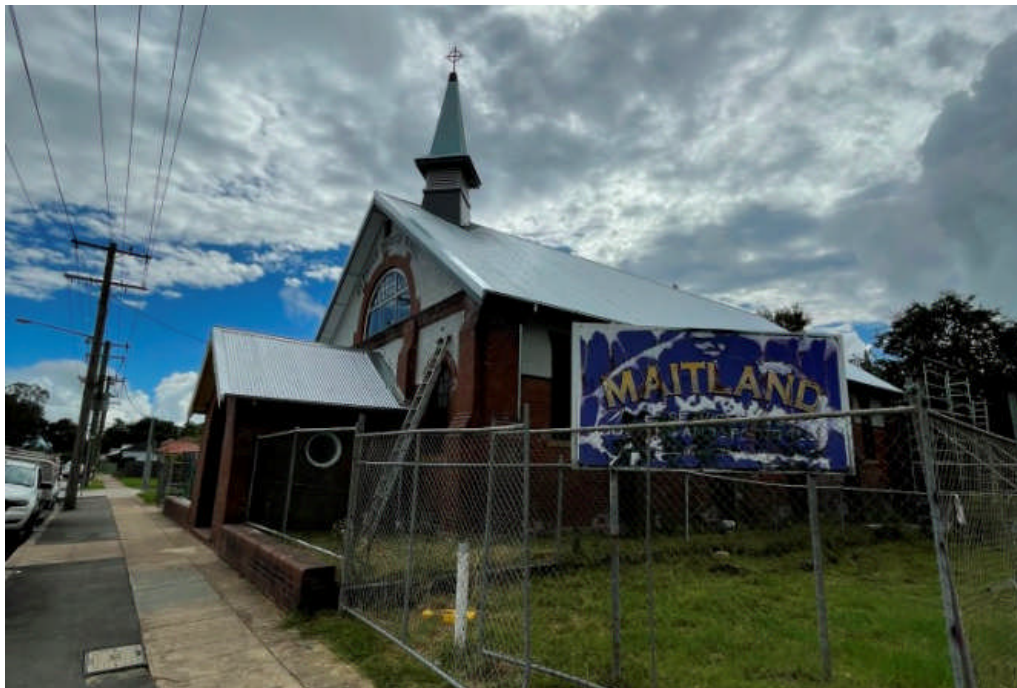
Plate 8: St Pauls Parish Hall nearing completion of restoration works. (SHAC)
