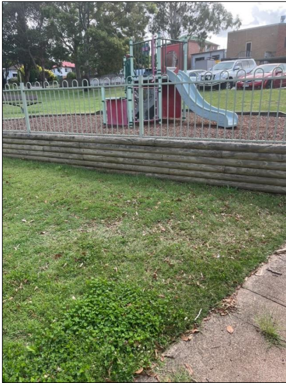
Figure 6: Cut and fill playground and retaining wall in the central-northern portion of site, facing north.
