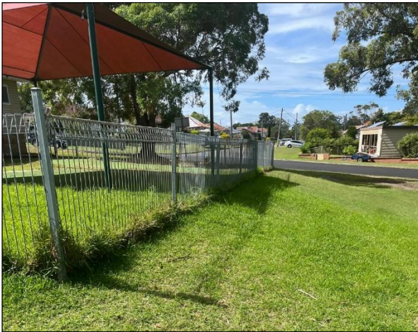
Figure 4: Fill pad area with an awning structure and fenced off area behind the community centre on the eastern side of the site. Facing east towards Tyrell St.
