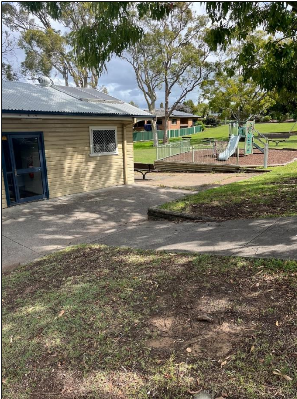
Figure 2: Community Hall in the central north-eastern portion of the site, looking south-west
