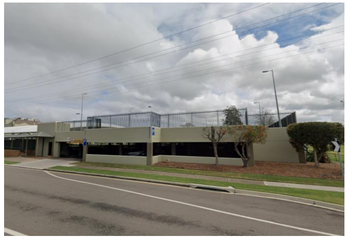
Figure 11: Club multi deck car park (source: Google Street view Sept 2020)
