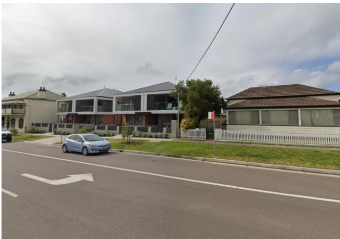
Figure 21: Existing residential buildings on opposite side Banks Street (source: google street view May 2021)
