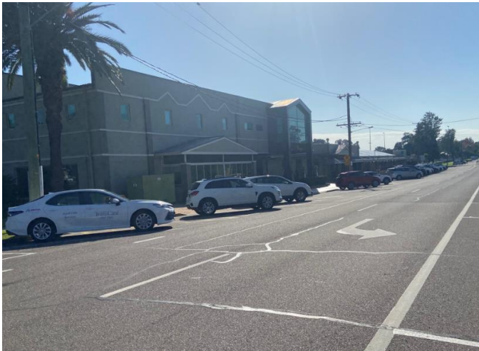
Figure 30: Street view from corner of Banks Street (source: author)
