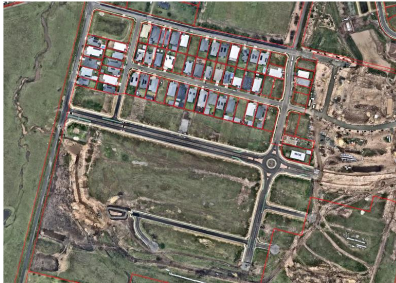
Figure 1 – Aerial view of the site (Source: Nearmap 2024)
