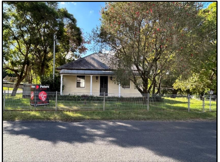
Photo 2: Existing dwelling fronting Bayswater Road
