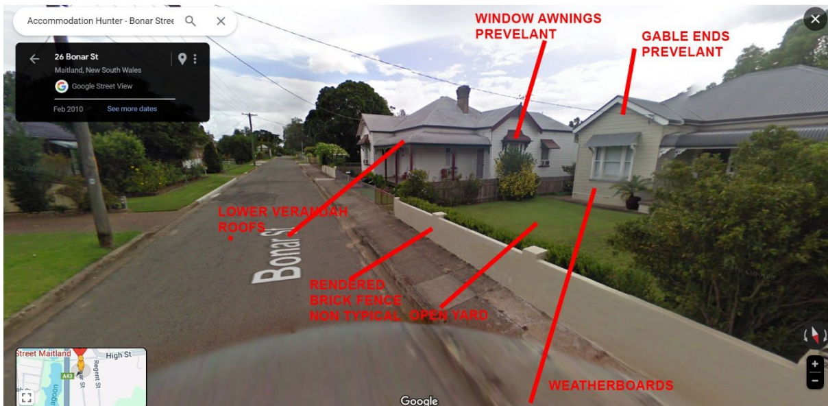
Figure 18 - View of Bonar Street Looking south. Victorian styled homes with gable ends, window awnings, double hung windows. Separate verandah roofs. High pitched roofs. Varied setbacks along length of street some homes being close to street 1 or 2m and others setback 5-6m
