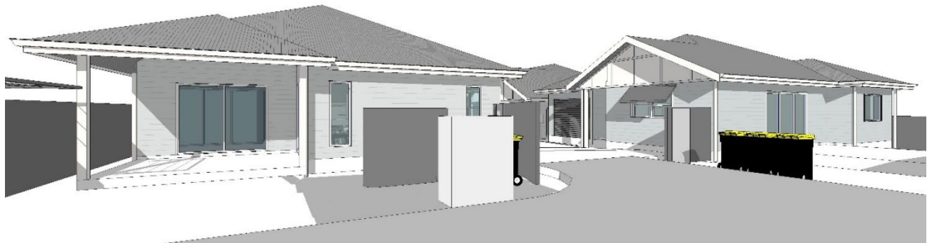
Figure 22: View of Dwellings with fences taken out looking south. Traditional hip and gable roof forms. Gables have detailed trims. Double Hung Windows used to front facades with window awnings where required. Weatherboard cladding used in 2 x different colour tones.
