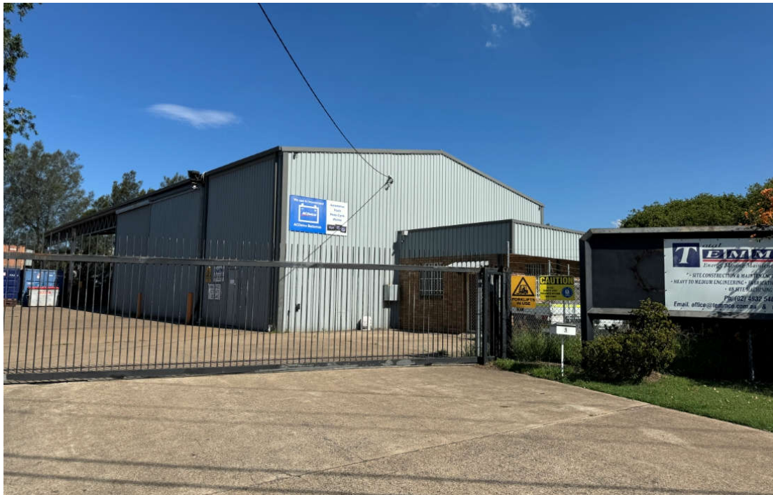
PHOTO 1 - SITE PHOTO LOOKING EAST
