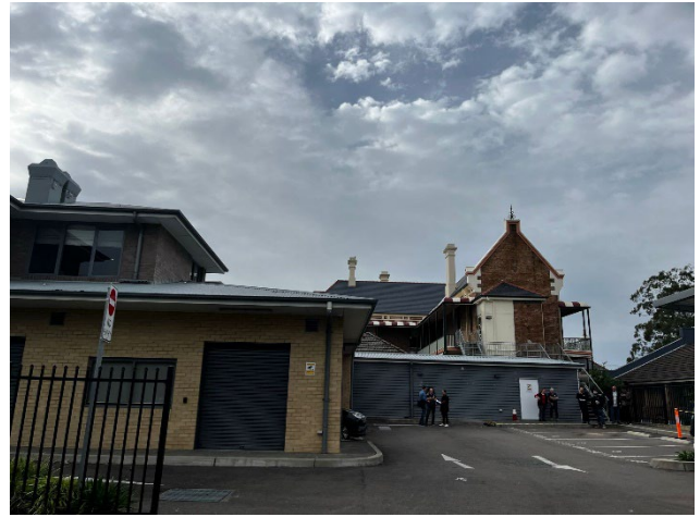
Picture 2 View of site from entrance on Bonar Street
