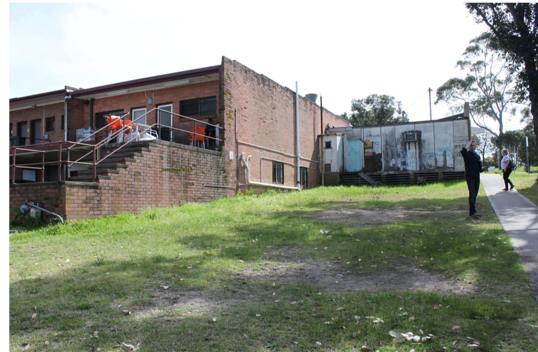
4. POOR OUTLOOK TO BACK OF SHOPS
