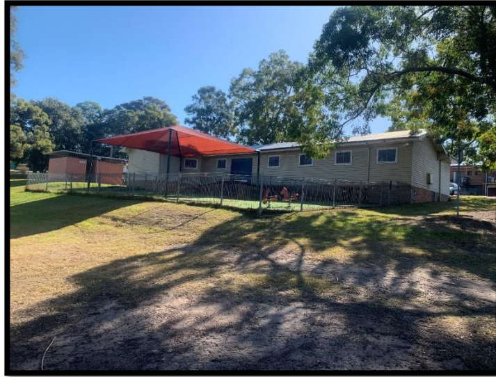
Figure 1 - Photograph of site
