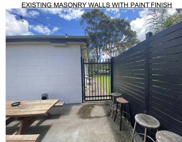
EXISTING MASONRY WALLS WITH PAINT FINISH
