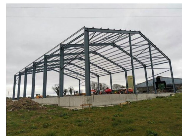
EXAMPLE OF STEEL PORTAL FRAME
