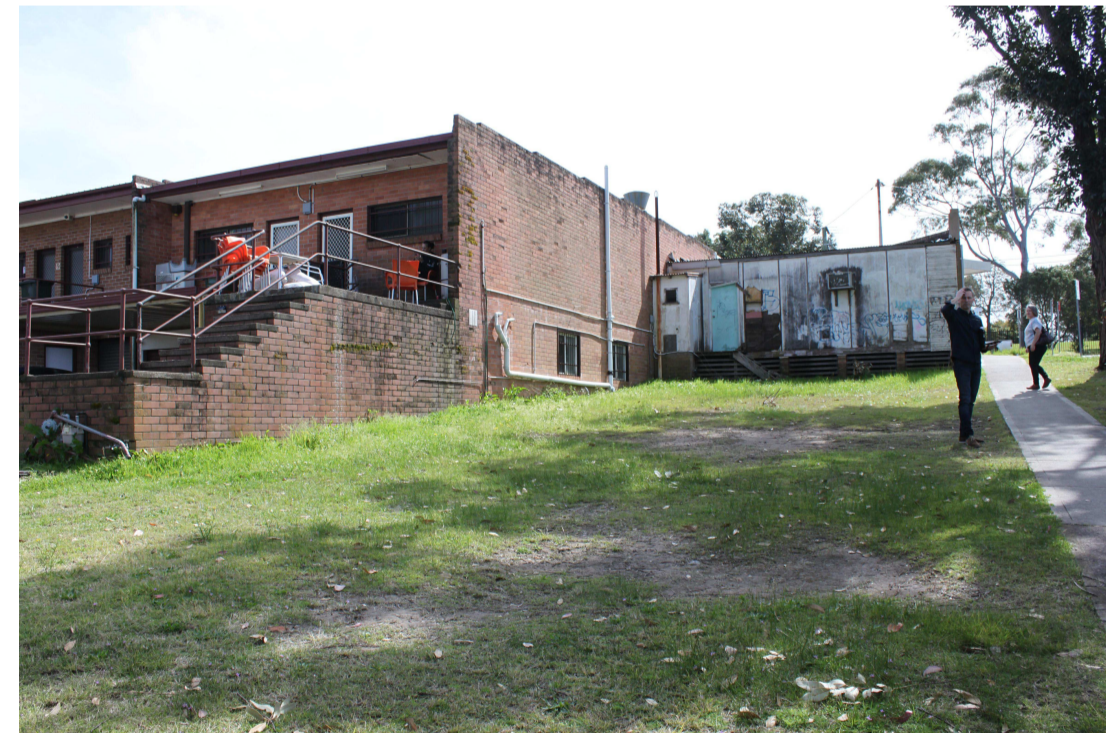
4. POOR OUTLOOK TO BACK OF SHOPS
