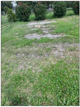
Figure E24: placed fill, comprising crushed concrete, tile and brick in the southern portion of Lot 7, looking south-west
