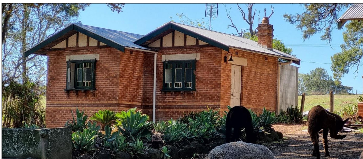
Figure 4: Existing Coach House and Studio
