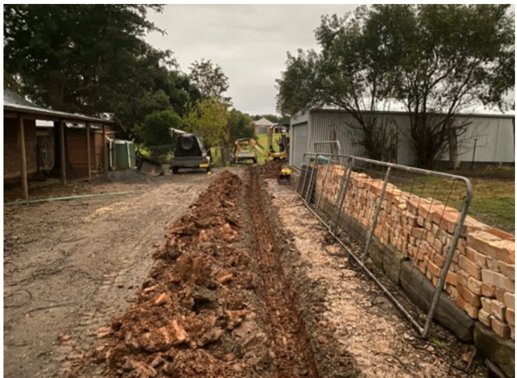
Plate 20 – Photo showing drainage works and new shed to rear of the former Coach House. The bricks on the rhs were re-used on site (source: Craig Favelle).
