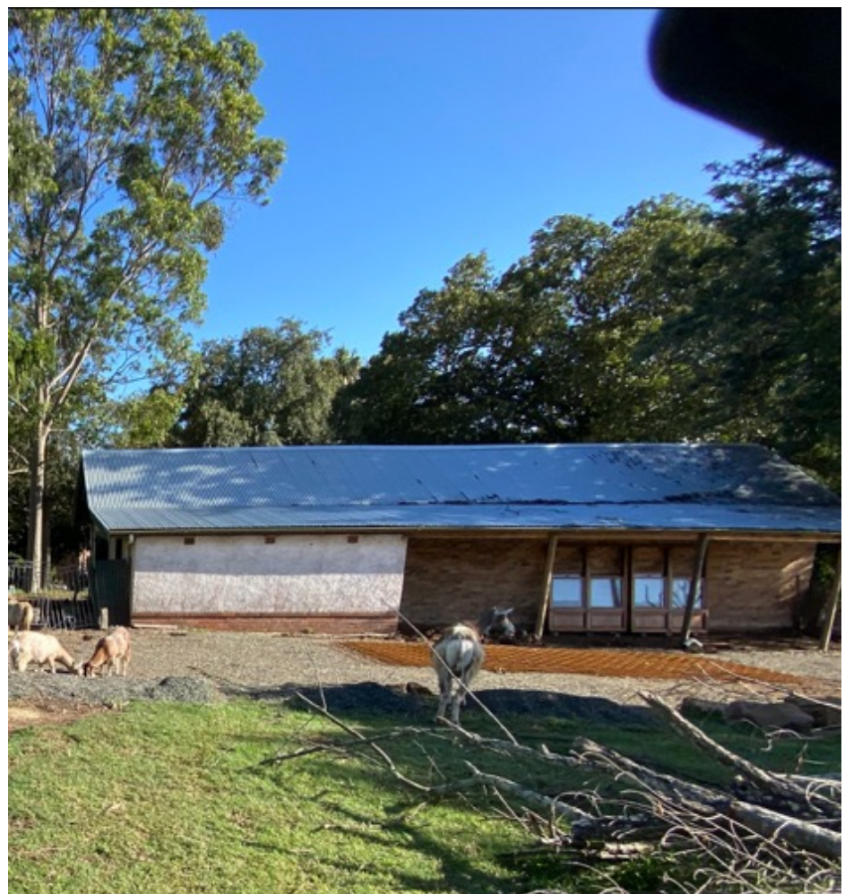
Plate 5 – Before photo showing works in progress for new deck at rear of former Coach House. Part of the brick work on the south elevation was removed to install new windows and doors (source: Craig Favelle).
