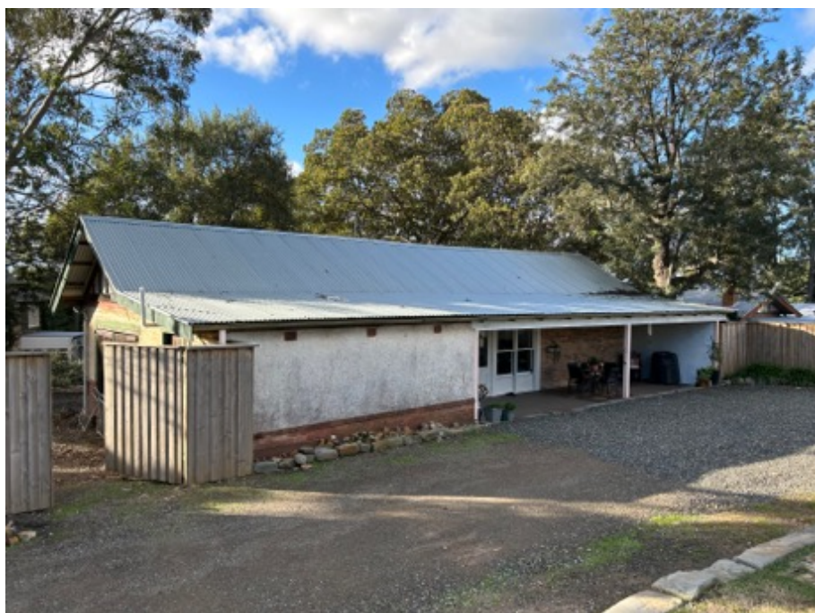
Plate 7 – Close up photo showing the new deck with windows and doors added to the rear of the former Coach House forming the main entry to the dwelling. The removed bricks were re-used as pavement outside entrance to Coach House (source: Eikos 8/05/24).
