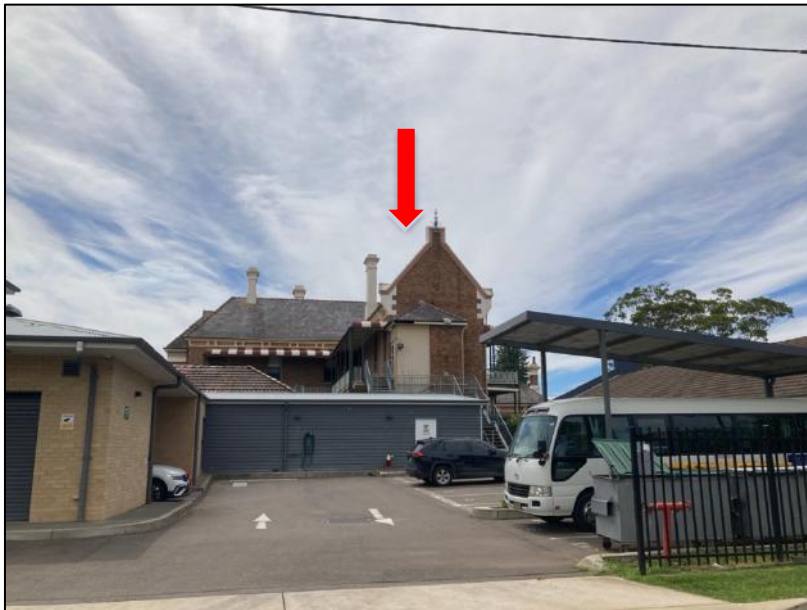
Figure 45: Looking east towards the rear of 'Benhome' from Bonar Street (View 4).
