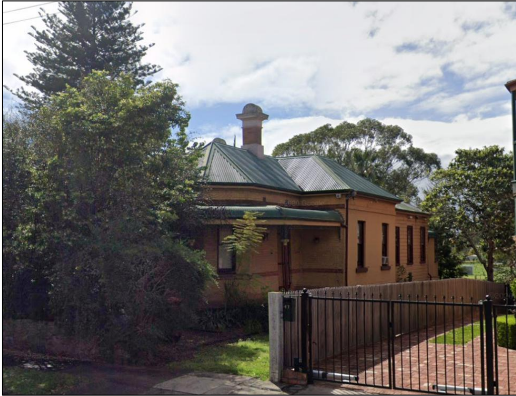
Figure 58: 'Victorian villa' as viewed from Regent Street.
