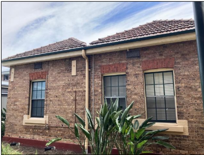
Figure 23: Eastern elevation of 'Dossie Cottage' (1B).
