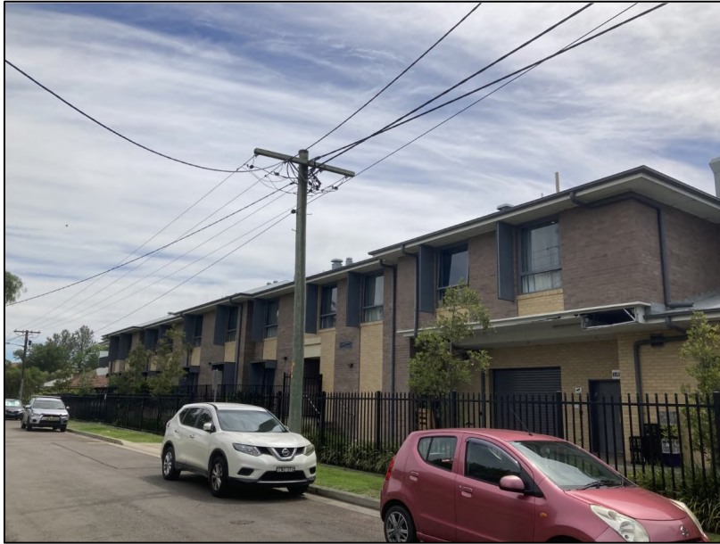
Figure 24: 'Benhome Board Building' (2) as viewed from Bonar Street.
