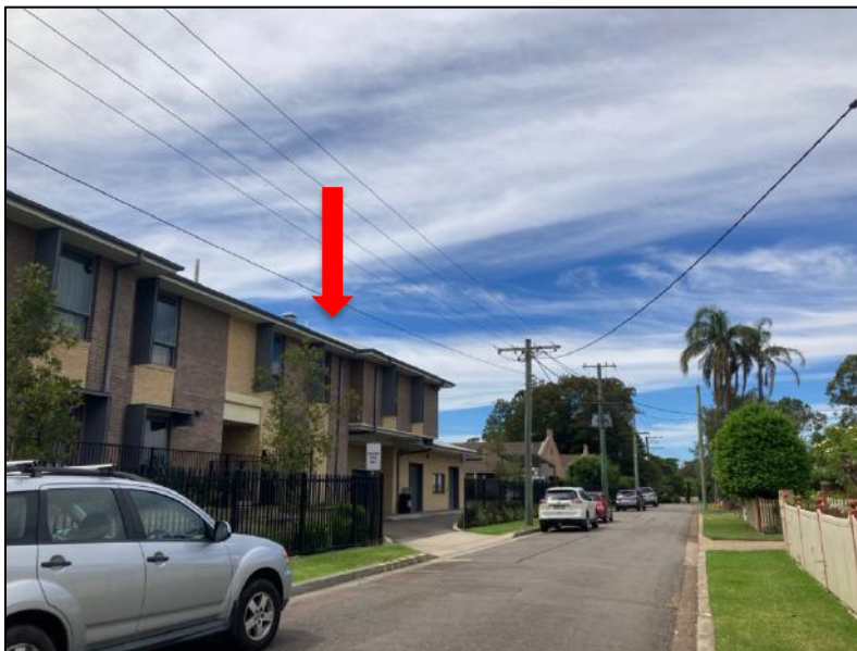
Figure 9: Bonar Street looking south. 'Benhome' is to the left as indicated by the red arrow.
