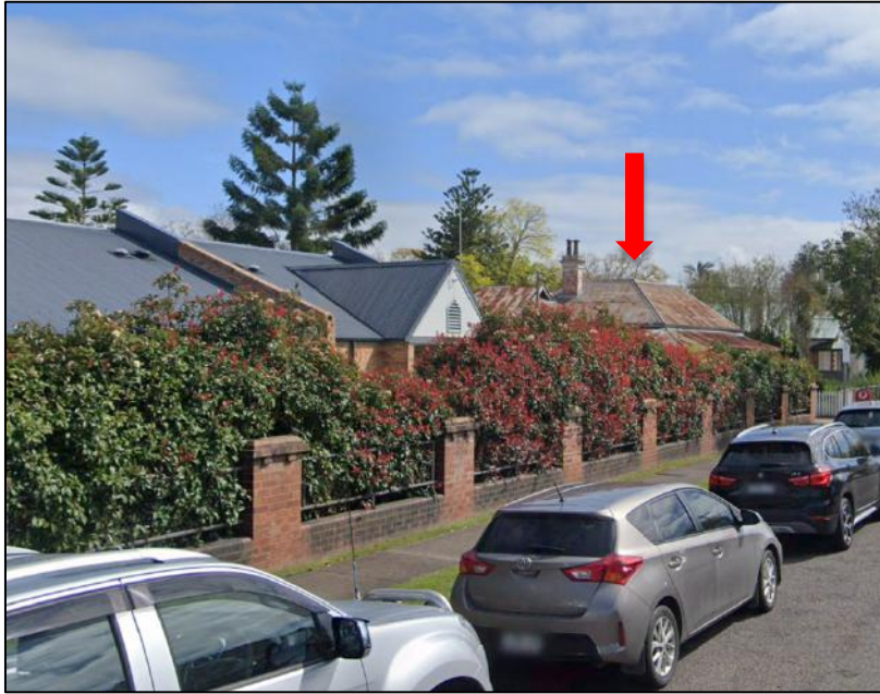
Figure 52: Looking towards the item on approach from the south on Regent Street (View 2).
