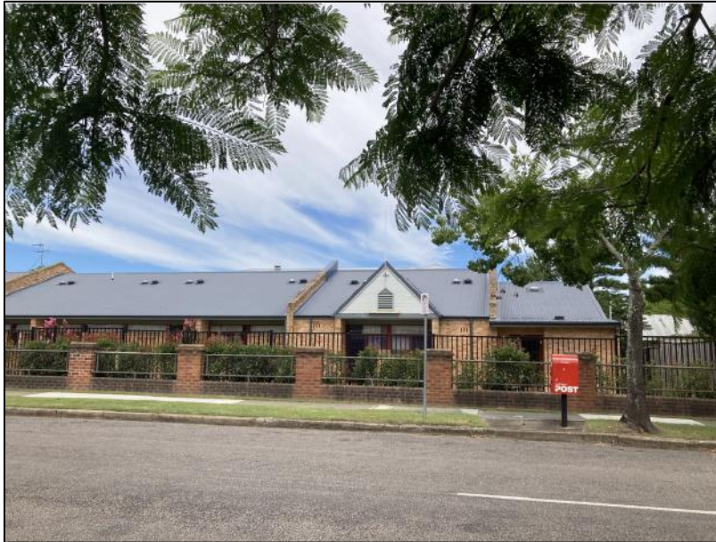
Figure 26: 'Rose Cottage' as viewed from Regent Street.
