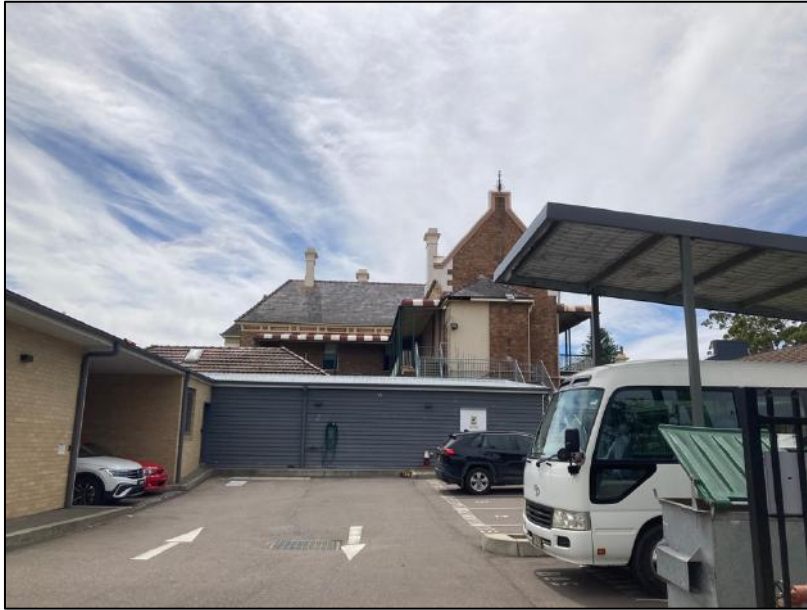
Figure 20: Rear elevation of 'Pender House' (1) showing a contemporary steel staircase. The 'Benhome Board Building' (2) is visible to the left.
