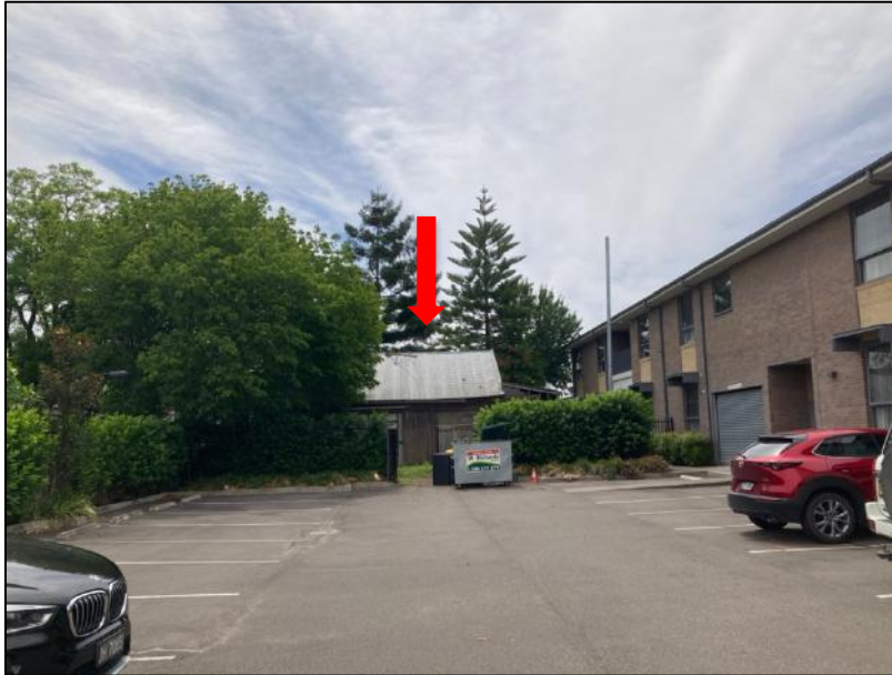
Figure 54: Looking towards the rear of the item from Bonar Street (View 4).
