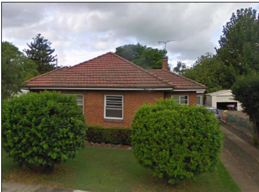
Figure 11: No. 13 Bonar Street to the north of the site, a single-storey mid-20 th century period dwelling.
