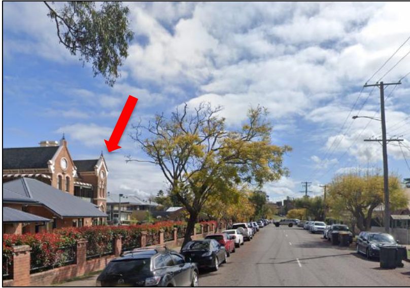
Figure 4: Regent Street, looking north. 'Benhome' is to the left as indicated by the red arrow.
