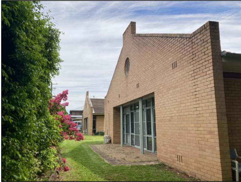
Figure 30: Looking obliquely across the front elevation of 'Curtis Wing' (5).
