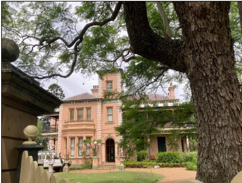
Figure 5: No. 35 Regent Street to the south of the site, a two-storey Victorian period dwelling.
