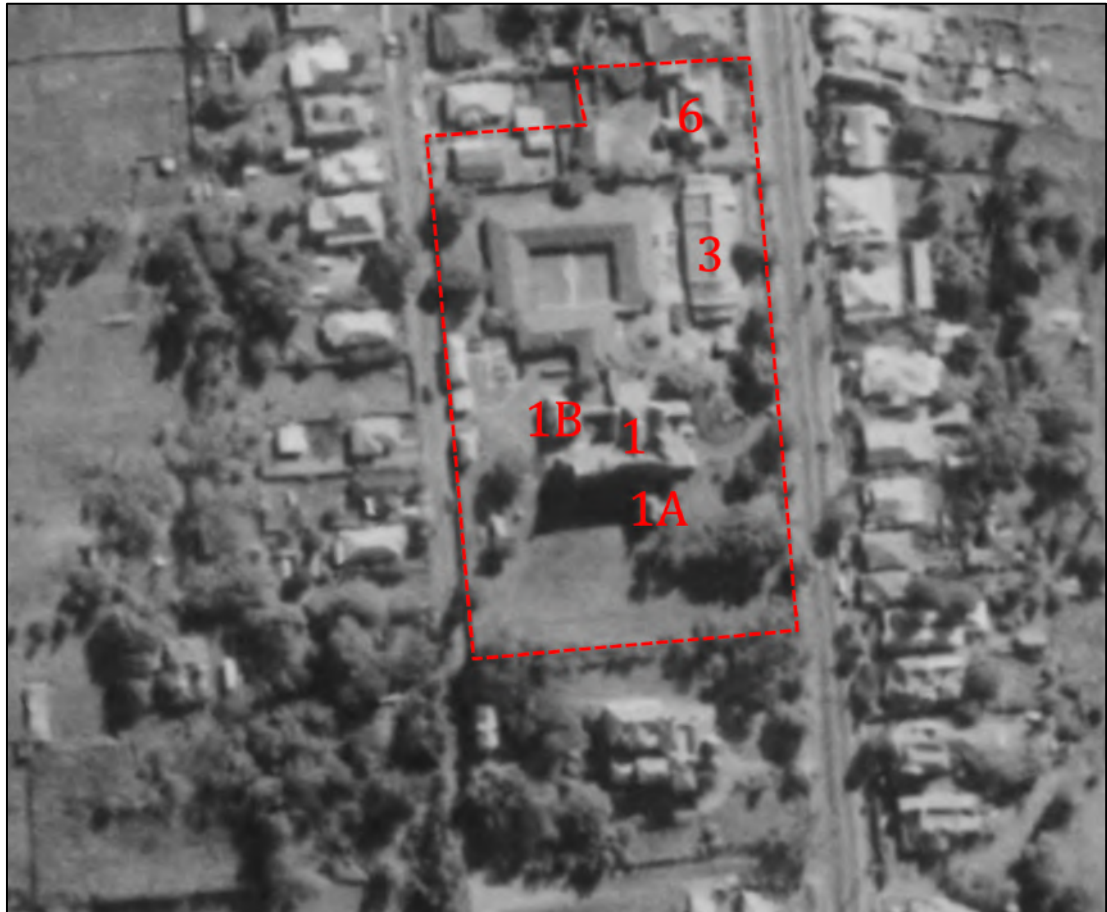
Figure 37: C. 1984 aerial photograph over the site. The current site boundaries are outlined in red.
