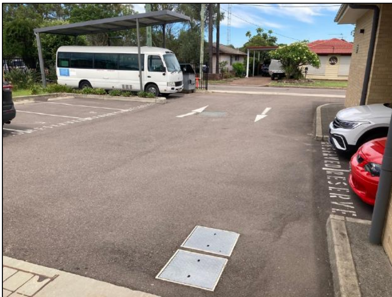
Figure 16: Parking area on the south side of the RFBI Benhome Masonic Village entry/exit via Bonar Street. A new extension is proposed in this area. The 'Benhome Board Building' (2) is visible to the right.
