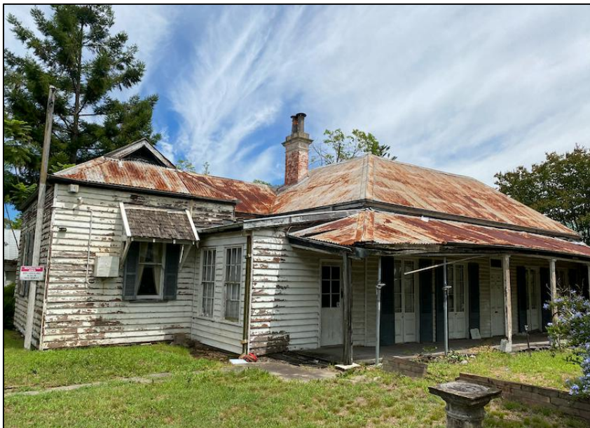
Figure 31: The front elevation of the heritage item 'House'.
