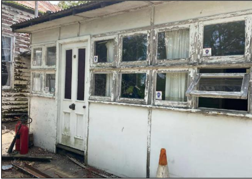
Figure 32: The rear elevation of the dwelling showing the later fibro enclosure.
