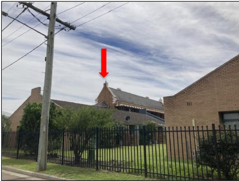
Figure 47: Looking towards the rear of 'Benhome' on approach from the south on Bonar Street (View 6).
