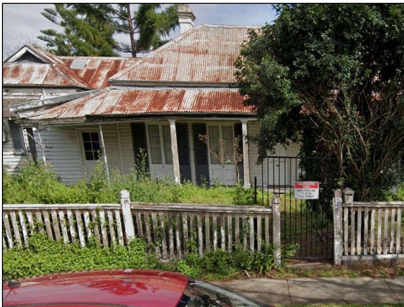
Figure 51: Looking towards the item from directly outside on Regent Street (View 1).
