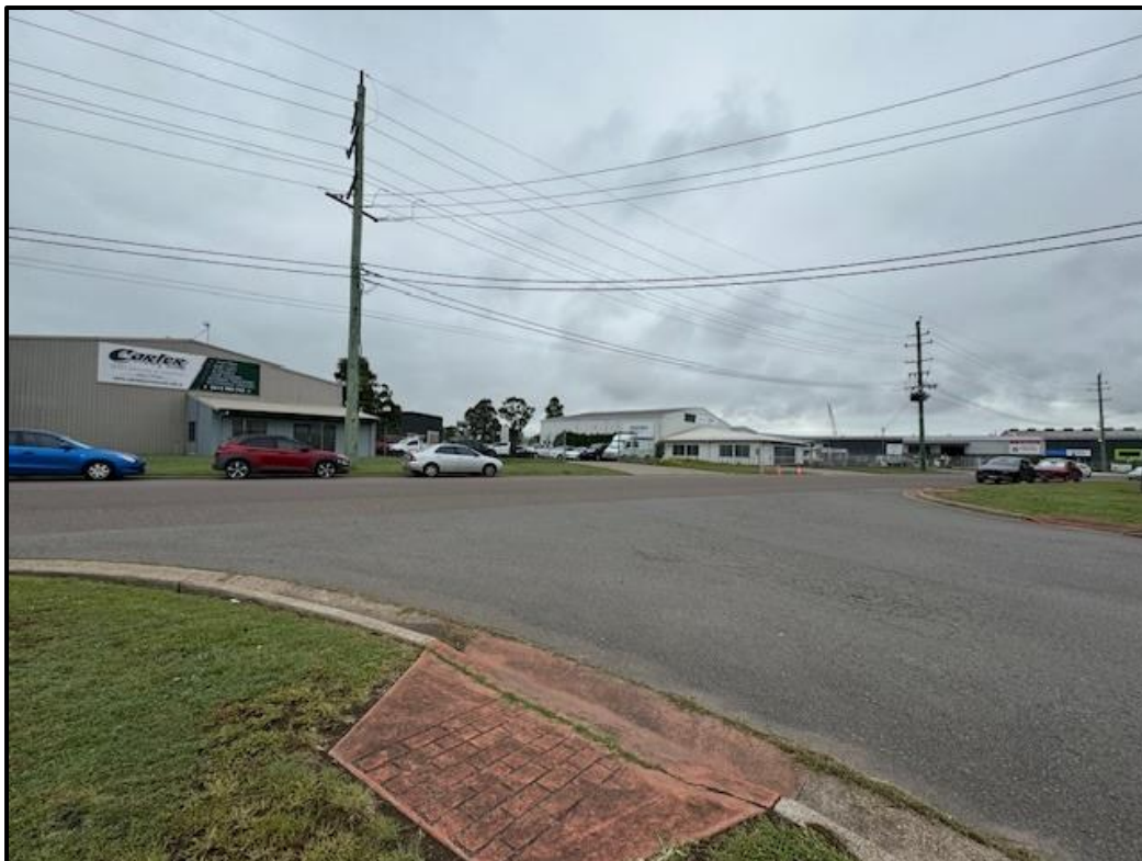
Photo 4 – Intersection of Burlington Place and Racecourse Road
