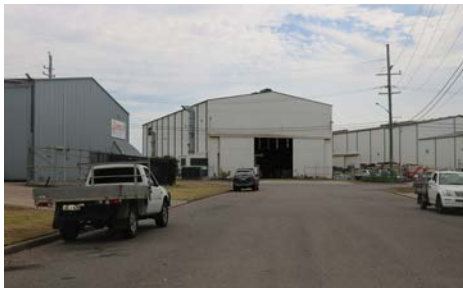
Image 6 Industrial warehouse within E4 Zone along Racecourse Road.
