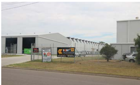
Image 10 Industrial warehouses within E4 Zone along Racecourse Road.
