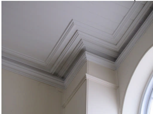
Plate 4.12: Timber lining board ceiling and cornice.
