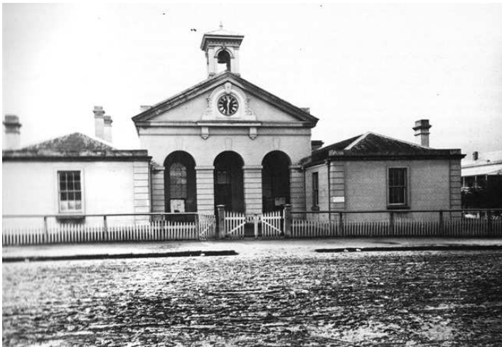
Plate 4.11: Armidale Court House constructed in 1860 with the Porch added in 1870.
