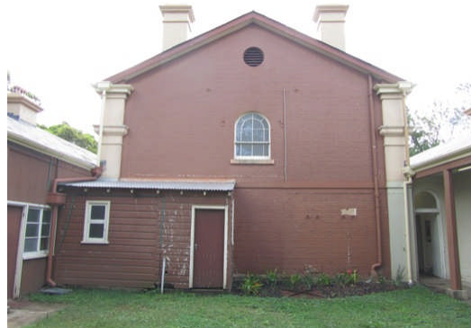
Plate 4.2: The southern courtyard and Bathroom.
