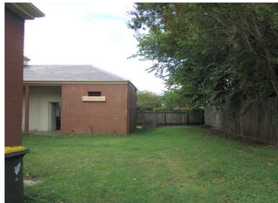
Plate 6.4: View from the Northumberland St. entry across the site of the demolished Stables.
