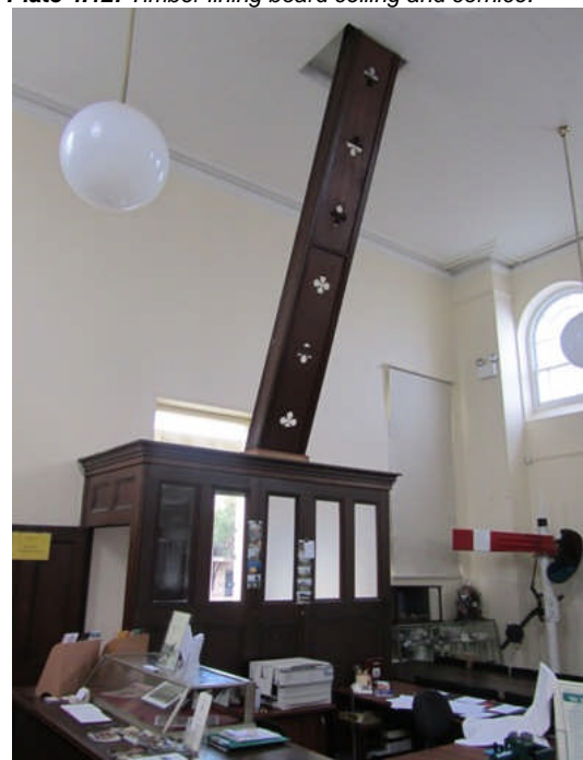
Plate 4.14: Timber Windlock and stair to clock in roof.
