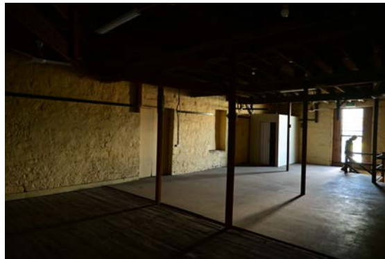
Figure 56: View of the southern elevation of the first floor.
