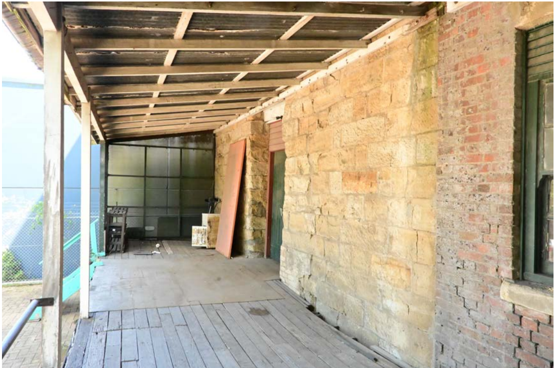
Figure 32: View of the rear elevation of No.101.
