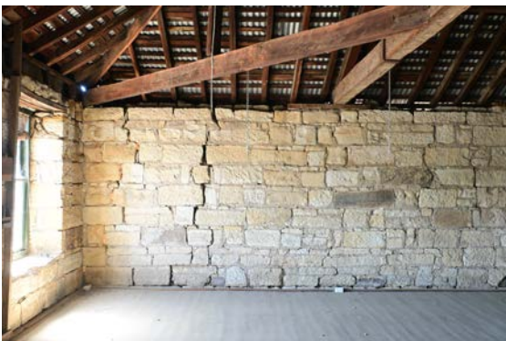
Figure 63: View of the top floor facing south.
