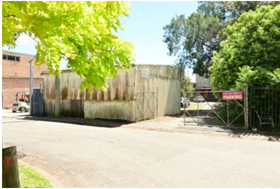
Figure 87: View northeast towards 'Smiths Flour Mill' from Mill Street.
