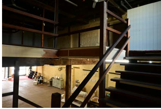
Figure 53: View of the internal stairs between ground and first floor.
