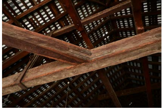
Figure 66: View of the roof framing at the front of the building.
