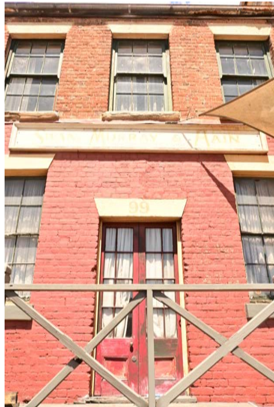
Figure 24: View of the front elevation of No.99.
