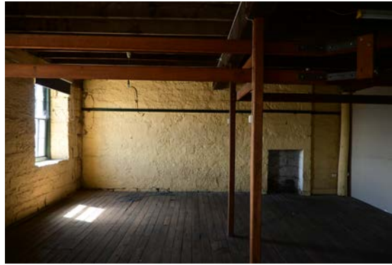
Figure 58: View of the first floor towards the front facing south.
