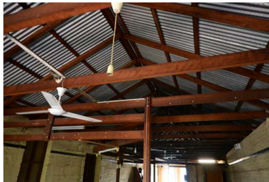
Figure 42: View of the exposed roof framing.
