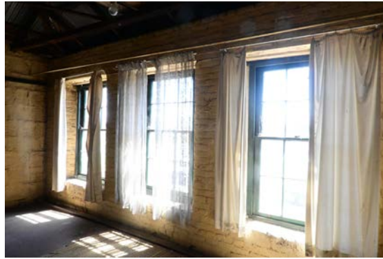
Figure 44: View of the rear elevation windows at the first floor.
