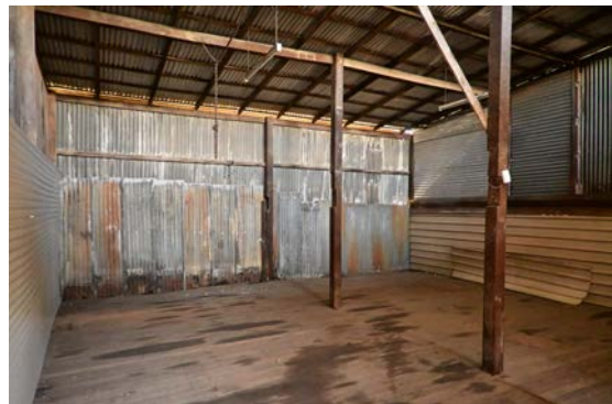
Figure 77: View of the shed interior.
