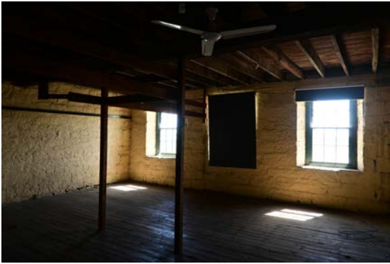
Figure 57: View of the first floor facing towards Newcastle Street.
