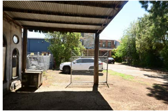
Figure 79: View of the annex to the rear shed.
