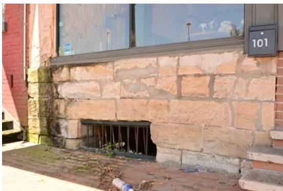
Figure 20: View of the left hand side of front entry to No.101.
