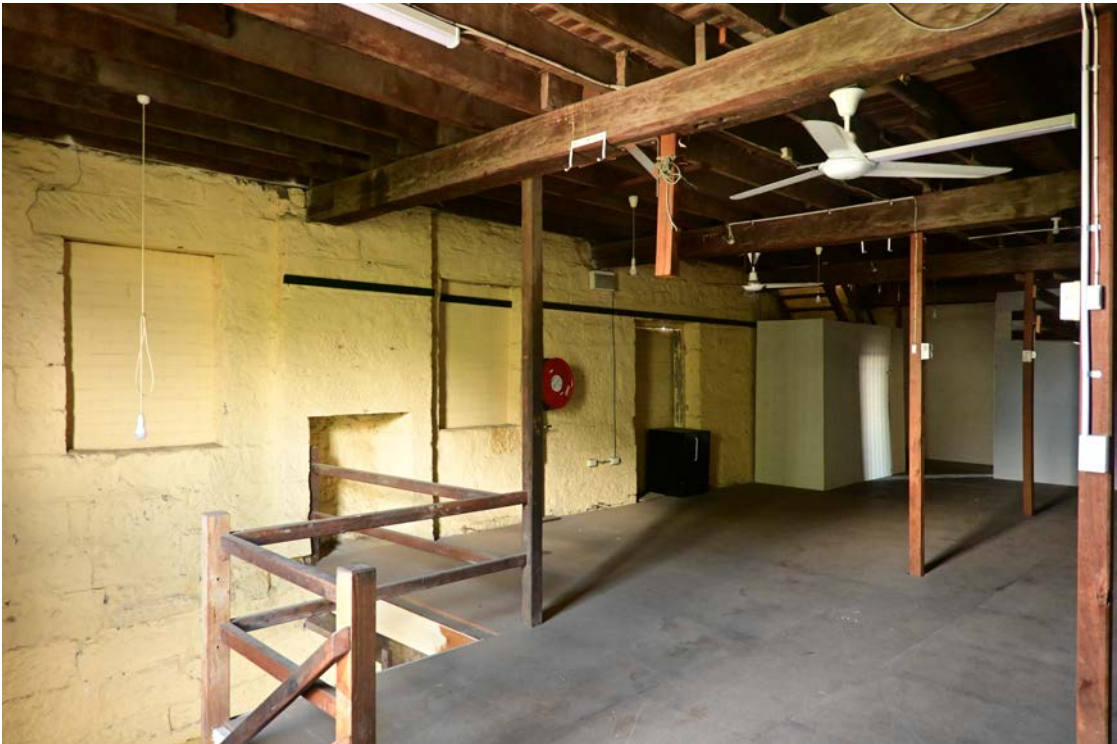
Figure 54: View of the first floor facing northeast.
