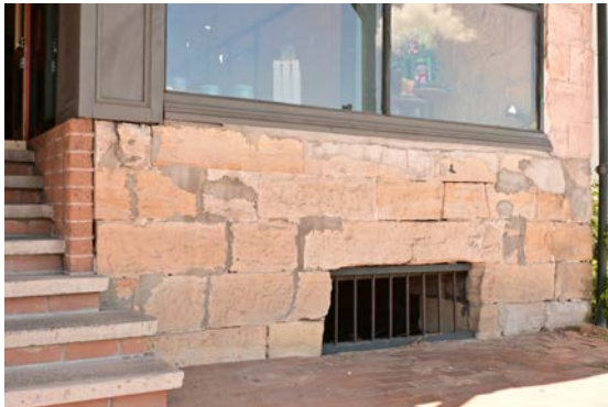
Figure 19: View of the right hand side of front entry to No.101.
