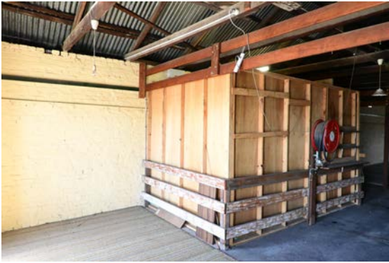
Figure 43: View of the partitions to the internal staircase at the first floor.
