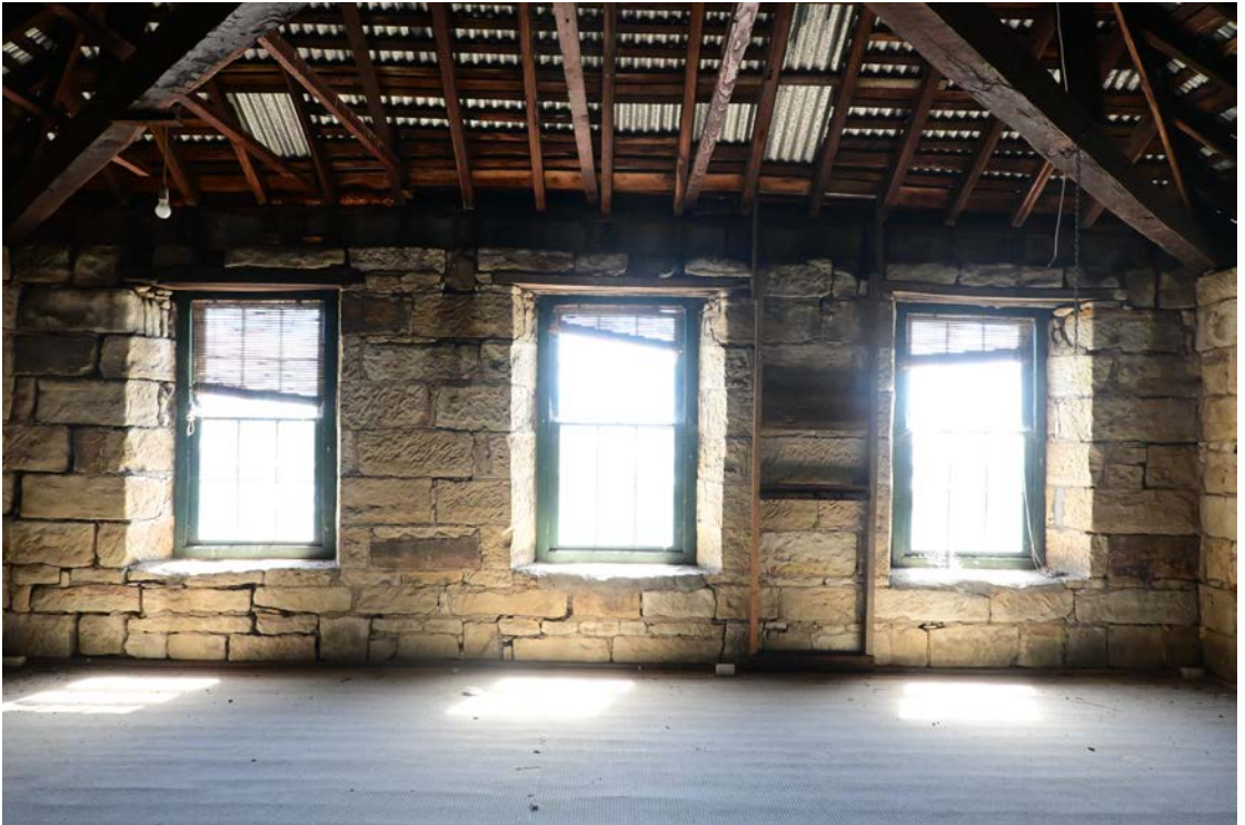
Figure 74: View of the top floor facing towards Newcastle Street.
