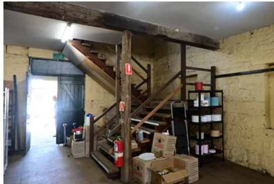
Figure 49: View of the ground floor staircase.
