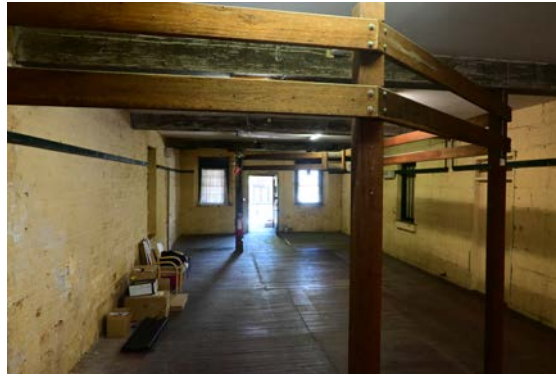
Figure 39: View of the ground floor facing towards the rear.
