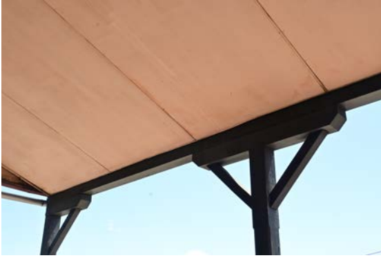
Figure 26: View of the front verandah post detailing.
