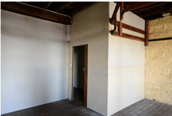
Figure 61: View of the first floor store room at the rear.
