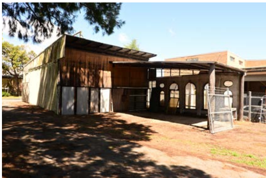
Figure 76: View of the rear shed.
