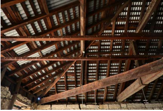
Figure 65: View of the roof framing at the front of the building.
