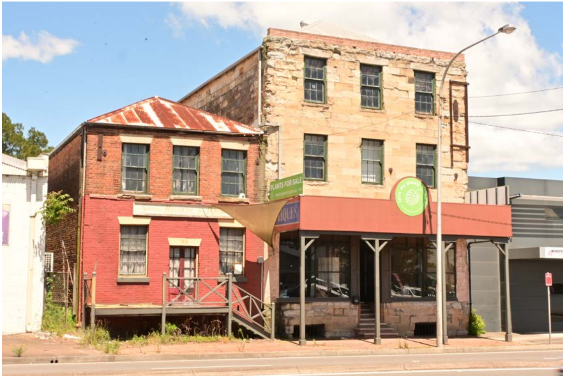
Figure 18: View of the buildings from Newcastle Street.
