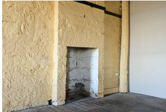
Figure 60: View of the first floor fireplace on the southern elevation.
