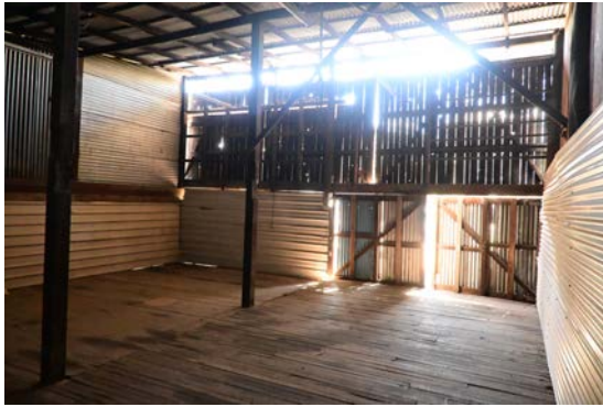
Figure 78: View of the shed interior.
