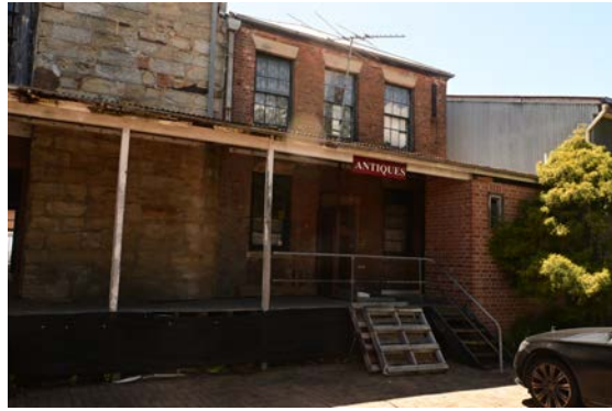
Figure 31: View of the rear elevation of No.99.
