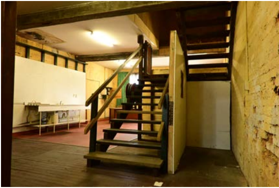
Figure 38: View of the ground floor staircase.
