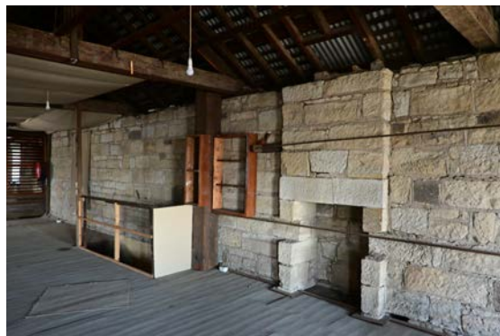
Figure 64: View of the top floor from the front facing northwest.
