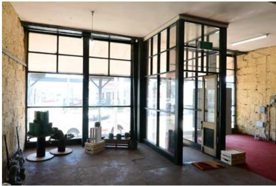
Figure 46: View of the ground floor main entry.
