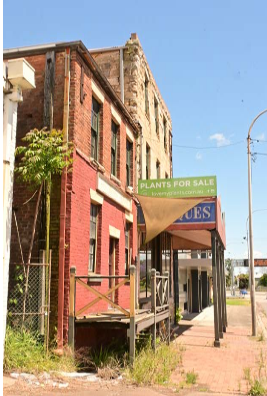
Figure 28: View of the front elevation.
