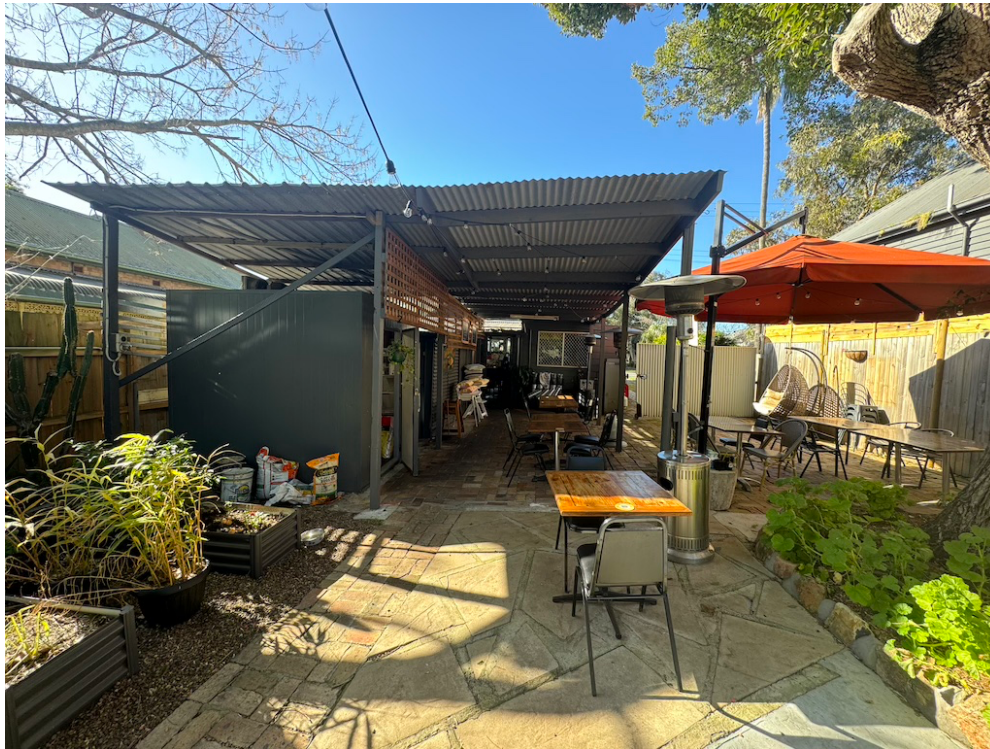
Figure 6 Rear structure to be demolished and rebuilt with masonry boundary wall
