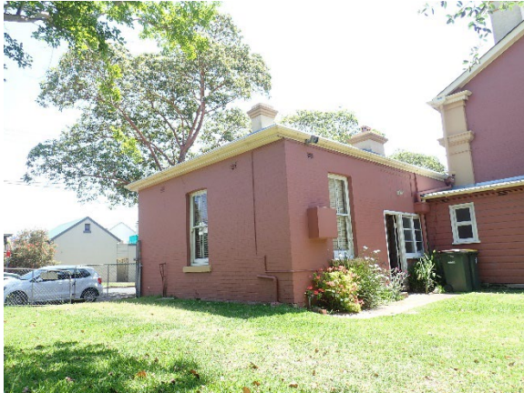
Image 5: rear kitchen wing Source: Placemark 01.11.2018
