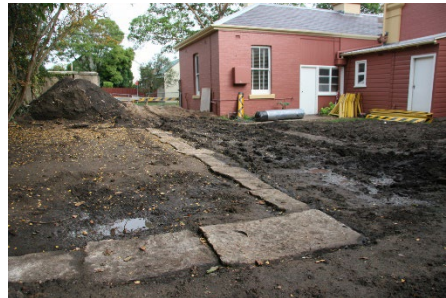
The Stables stone footings
