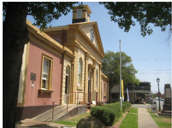
Image 14: Swan Street elevation & entry Source: Placemark 15.02.2018
