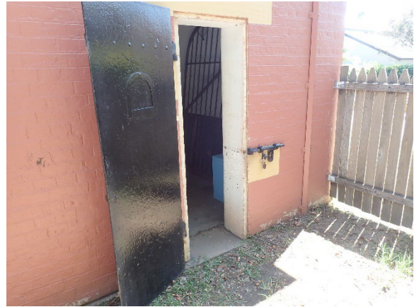
Image 12: side fence to cell block corner Source: Placemark 18.01.2019
