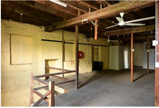
Figure 21: View of the first floor facing northeast.
