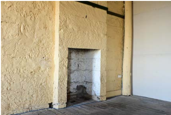
Figure 23: View of the first floor fireplace on the southern elevation.
