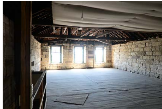
Figure 24: View of the second (top) floor facing southeast.
