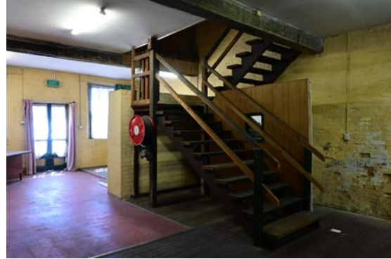
Figure 12: View of the ground floor staircase.
