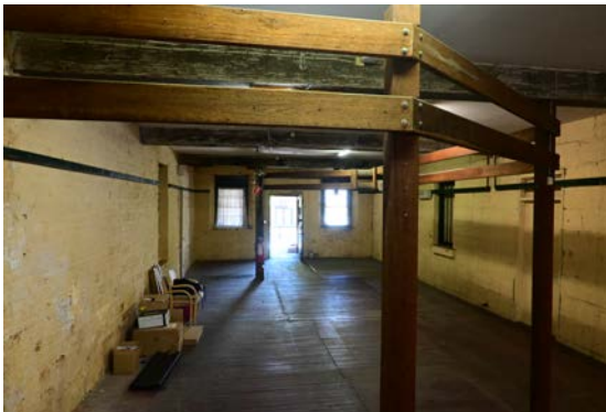
Figure 13: View of the ground floor facing towards the rear.
