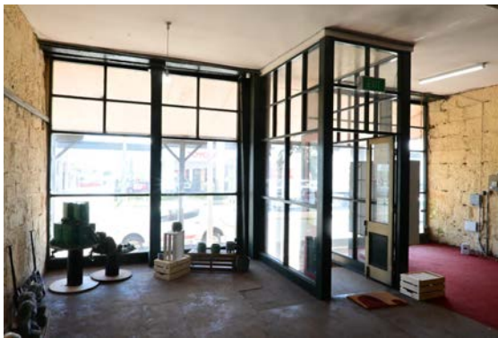
Figure 17: View of the ground floor main entry.
