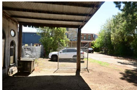
Figure 31: View of the annex to the rear shed.
