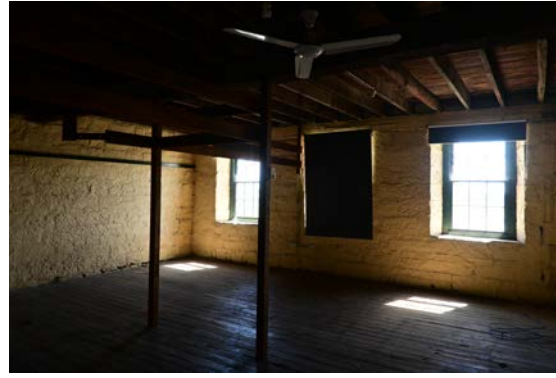
Figure 22: View of the first floor facing towards Newcastle Street.
