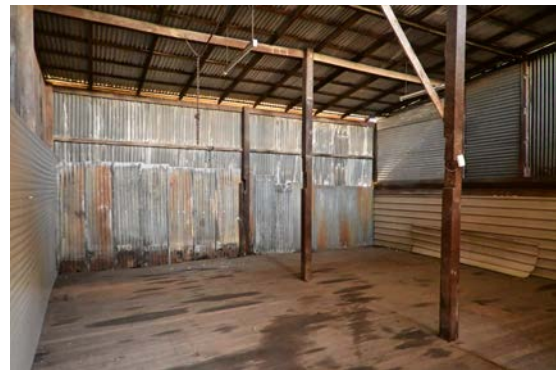
Figure 29: View of the shed interior.
