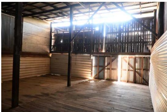
Figure 30: View of the shed interior.
