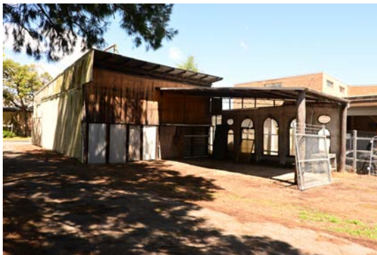
Figure 28: View of the rear shed.
