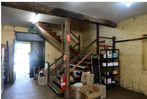
Figure 19: View of the ground floor staircase.
