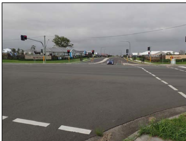
Figure 6.6 Intersection of New England Highway and Wyndella Rd
