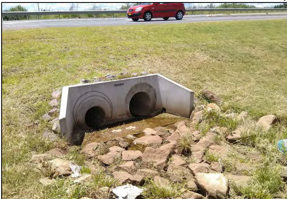
Figure 10 - Circular culverts beneath the New England Highway. (Looking upstream)
