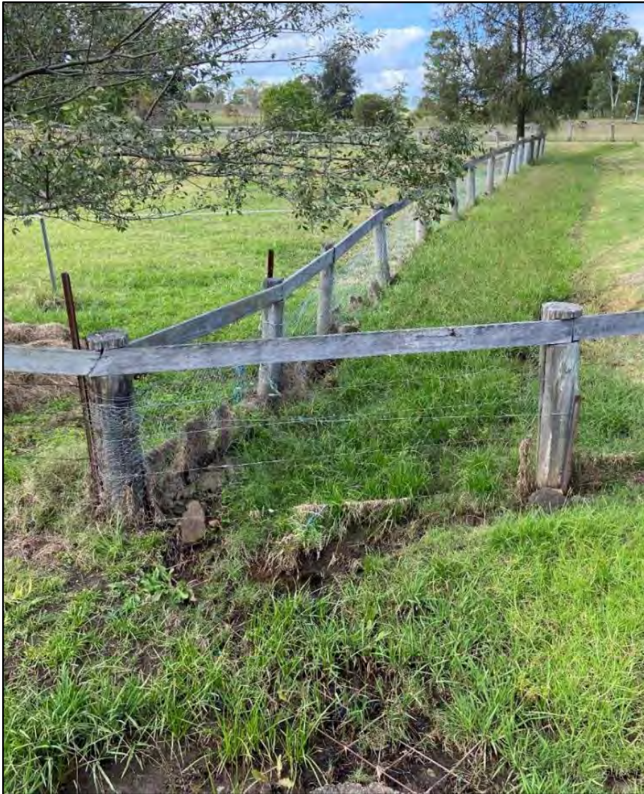
Survey Point 5.1 – mapped upstream
