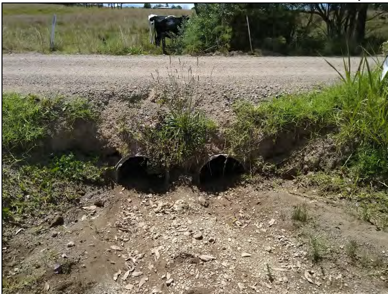
Figure 8 - Circular culverts beneath Wyndella Road. (Looking upstream)
