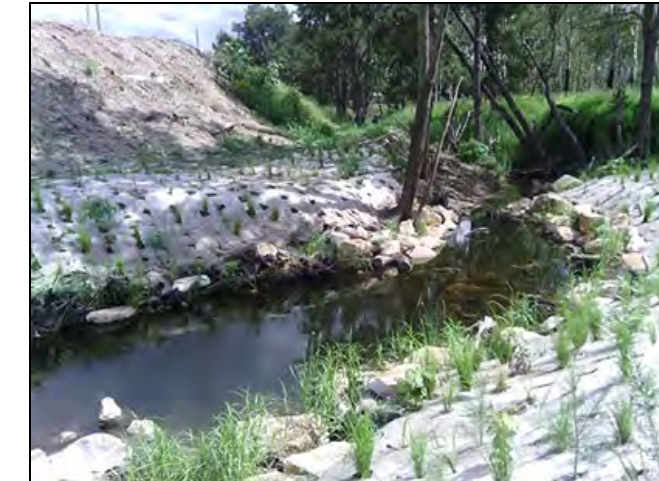
Plate 12 – Bundamba Creek Restoration works (Australian Wetland Consulting, 2018)
