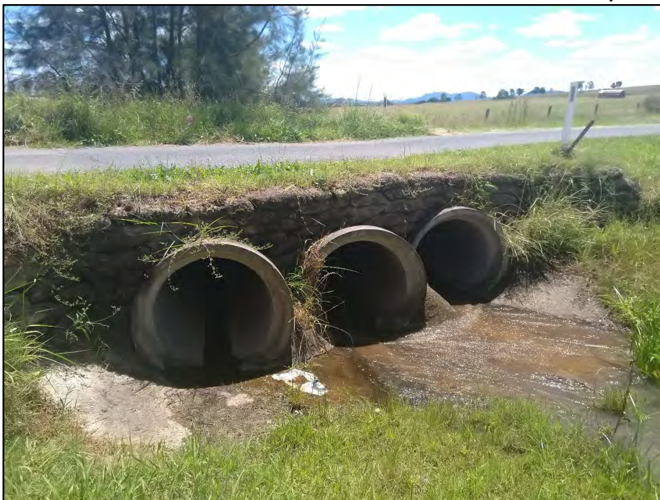
Figure 9 - Circular culverts beneath Wyndella Road. (Looking downstream)
