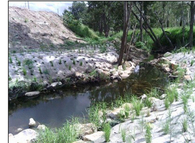
Plate 12 – Bundamba Creek Restoration works (Australian Wetland Consulting, 2018)
