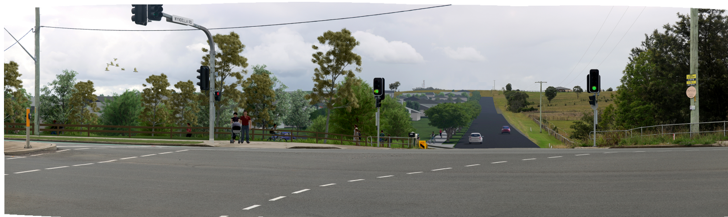
2. INDICATIVE DIGITAL MODEL AND PHOTOMONTAGE OF PROPOSED DEVELOPMENT ON SITE SHOWING SEVERAL YEARS GROWTH OF VMP-AREA AND STREET TREES. BILLBOARD KEPT FOR CONTEXT, BUT WOULD IN REALITY BE REMOVED FOR NEW SHARED PATH.
