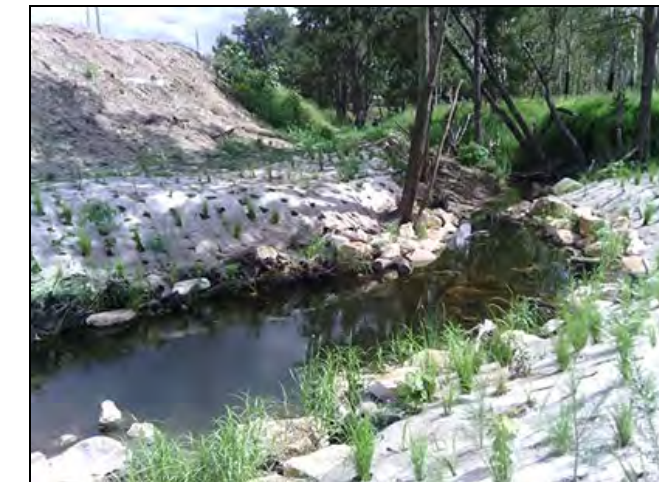
Plate 12 – Bundamba Creek Restoration works (Australian Wetland Consulting, 2018)
