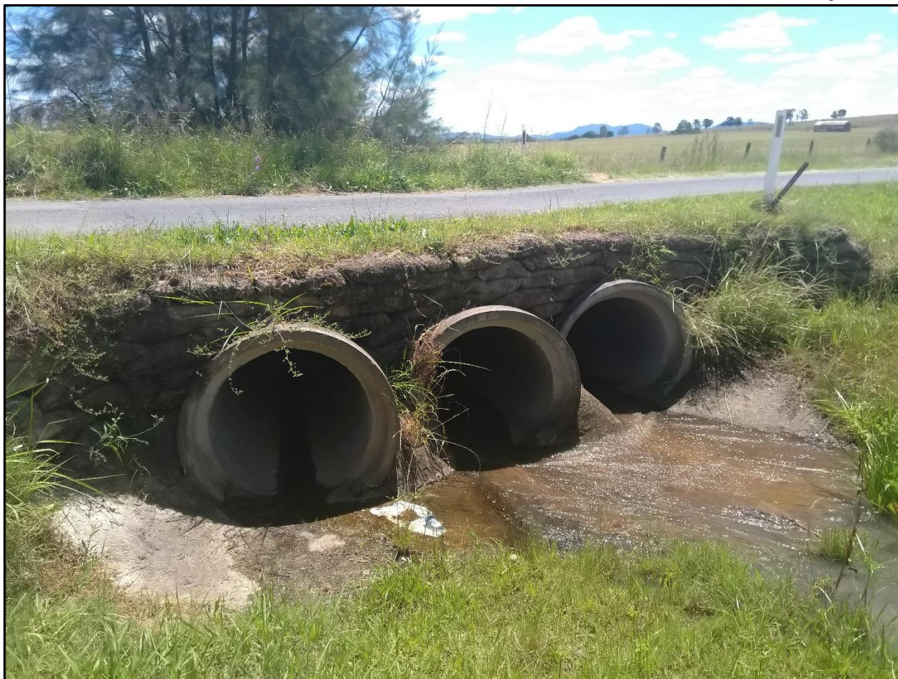
Figure 9 - Circular culverts beneath Wyndella Road. (Looking downstream)
