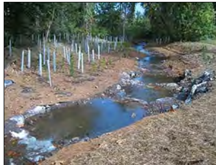
Plate 10 – Meanders, Riffles and shallow pools (STORMWATER, 2018).
