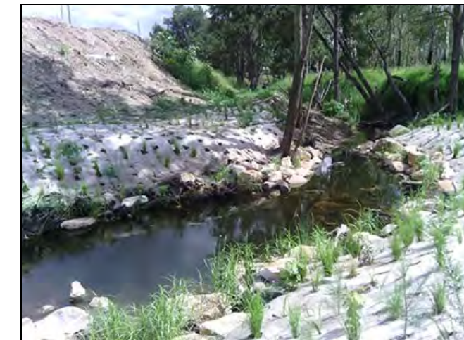
Plate 12 – Bundamba Creek Restoration works (Australian Wetland Consulting, 2018)
