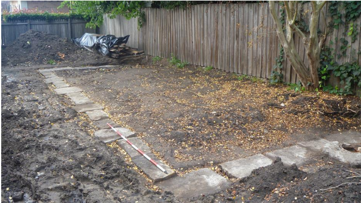
Figure 3.4 – Sandstone footings of the Police Stables, Morpeth Courthouse, facing south-east.
