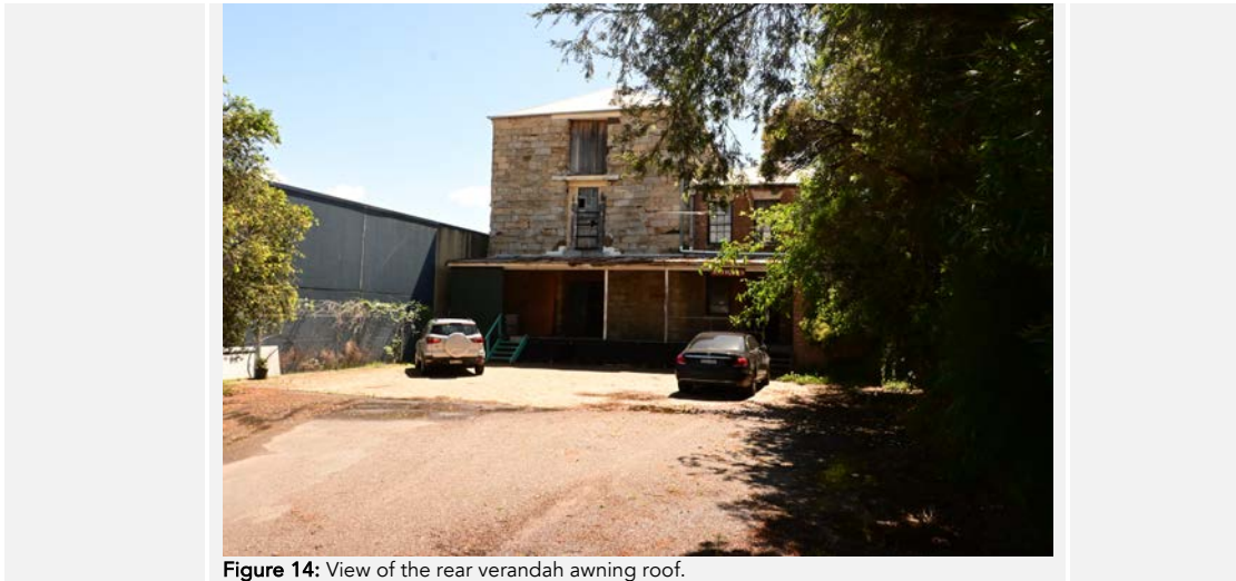
Figure 14: View of the rear verandah awning roof.
