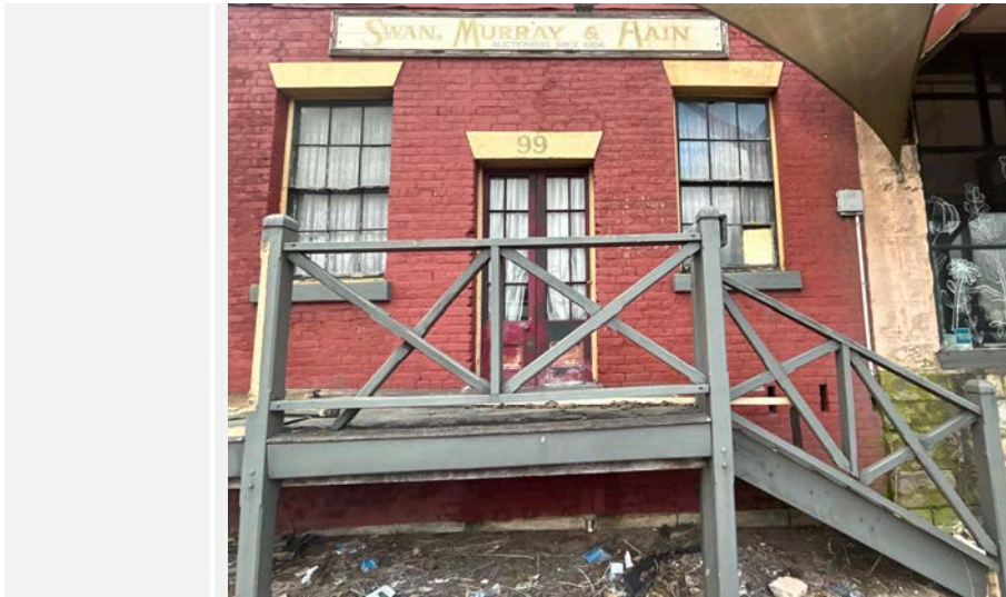
Figure 12: View of the front verandah.
