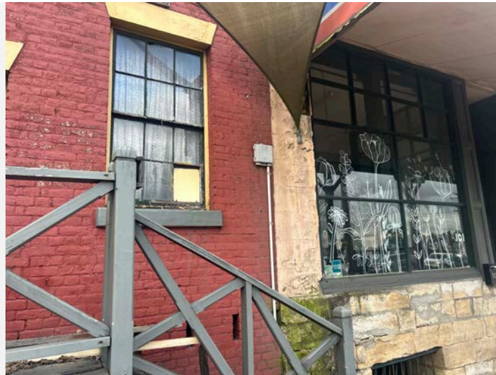
Figure 10: View of the existing telecommunications cabling at the front of the site.
