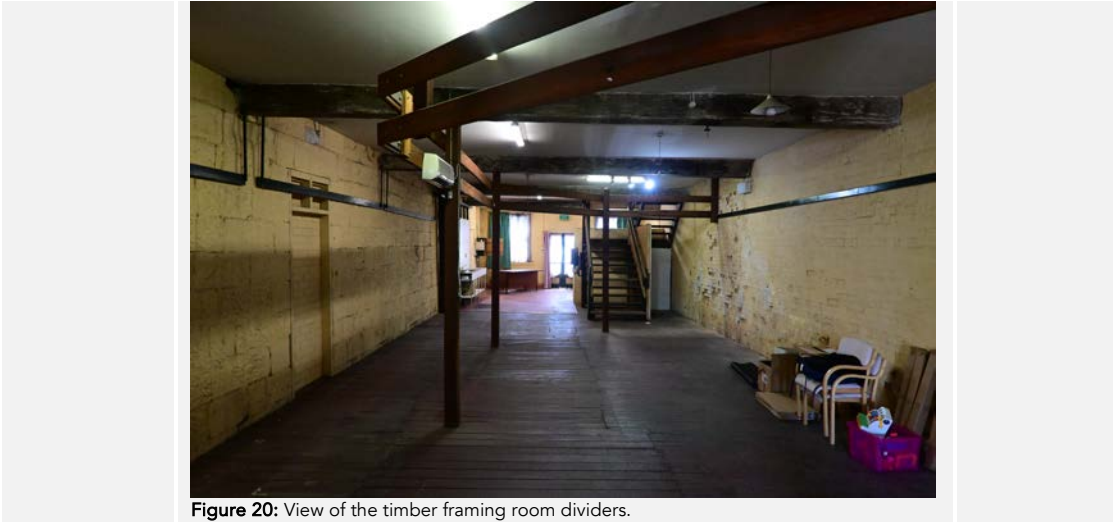
Figure 20: View of the timber framing room dividers.
