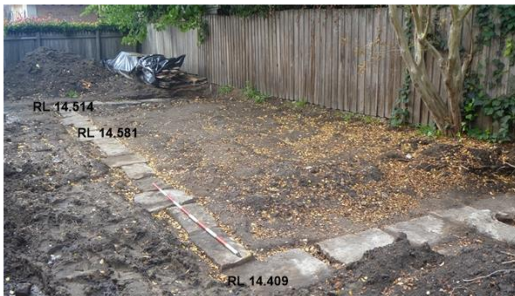
Figure 3.12 – Extent of sandstone footings of the c1862/63 Police Stables, At conclusion of 2013 excavation, looking south-east and showing RL taken in 2021.
