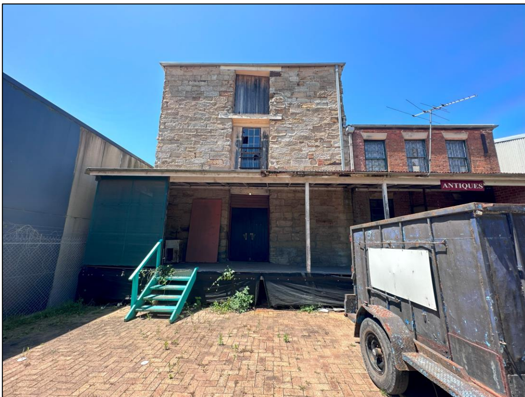
Image 6.2.1. View of the three-story sandstone commercial structure within the northern portion of the site, as observed from the central portion of the site on 10 November 2023, facing north-east.
