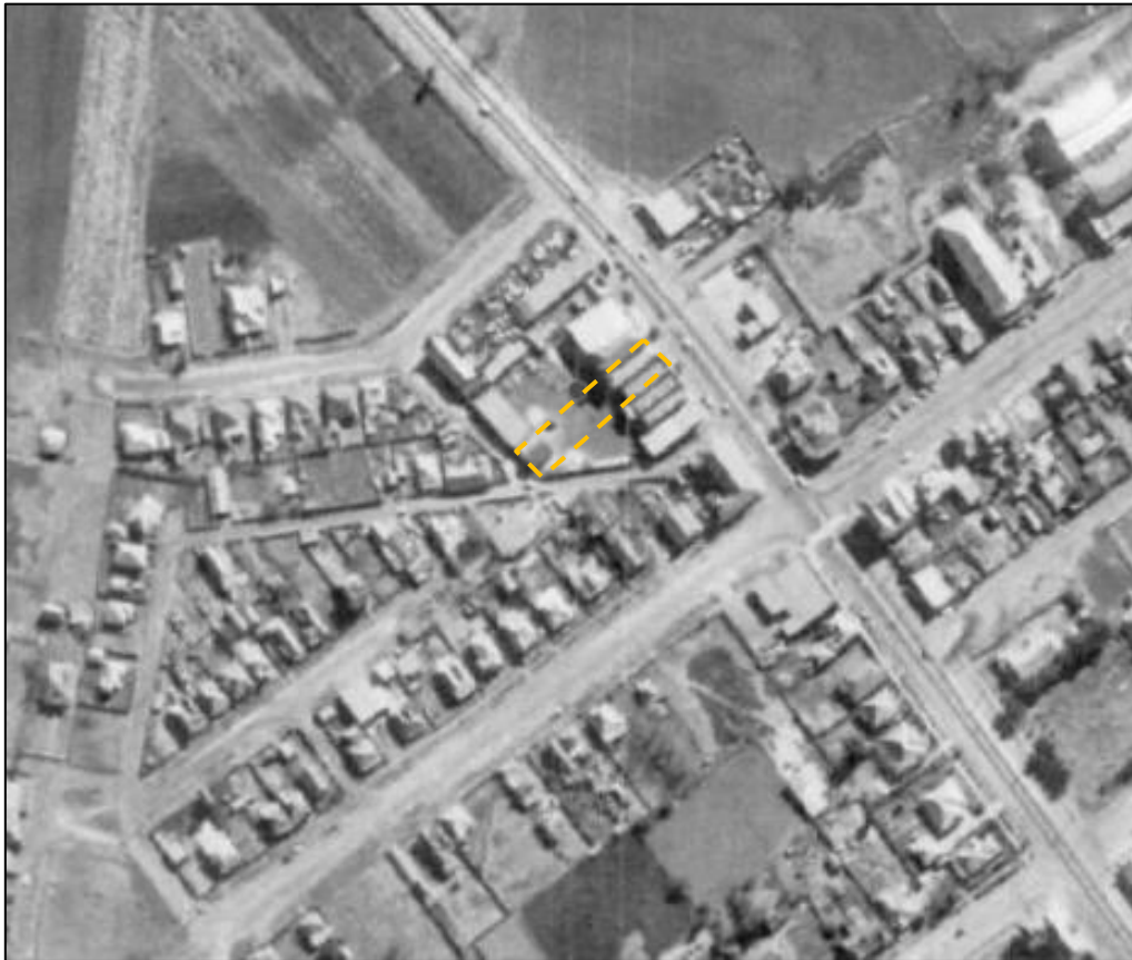
Historical Aerial Image 1: 1966 aerial image of the site.
