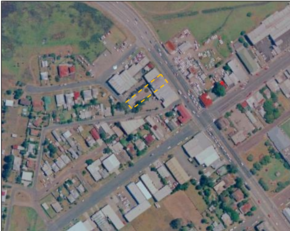
Historical Aerial Image 5: 2001 aerial image of the site.
