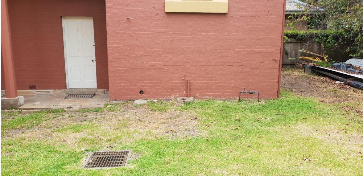
Existing stormwater pit in rear yard
