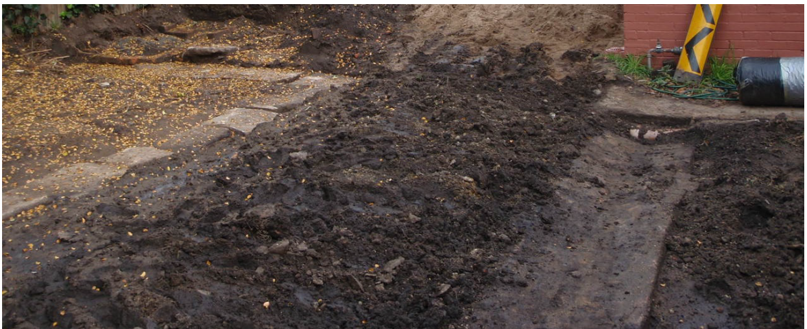
Old masonry dish drain (now buried) at right (kitchen wing in background), photo taken by archaeologist during excavation works 2014
