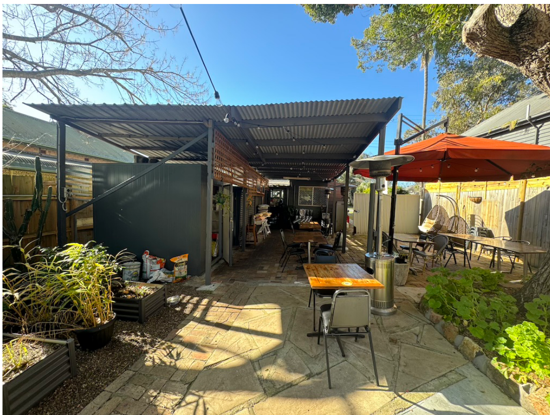
Figure 5 Rear structure to be demolished and rebuilt with masonry boundary wall
