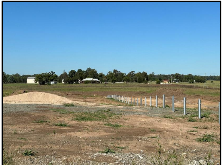
Photo 2: Subject site, as viewed from the north (across the drainage basin currently under construction)
