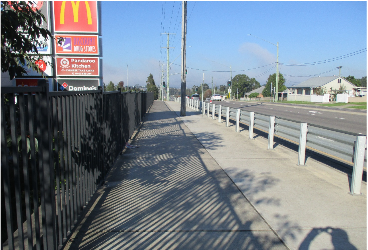
Photograph 8 – Off-road shared pathway eastern side of Cessnock Road.
