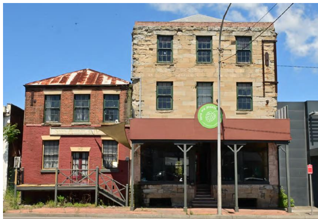
Figure 2-2: Existing Site fronting Newcastle St, East Maitland
