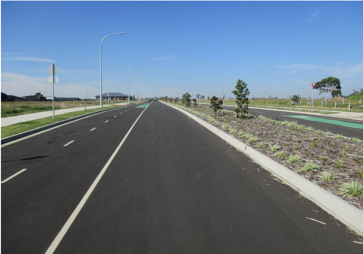
Photograph 7 – Springfield Drive near Station Lane.
