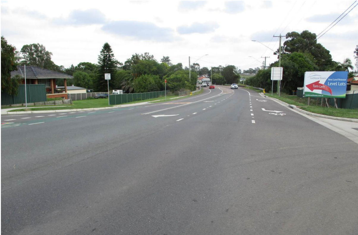
Photograph 3 – New England Highway near Station Lane intersection.
