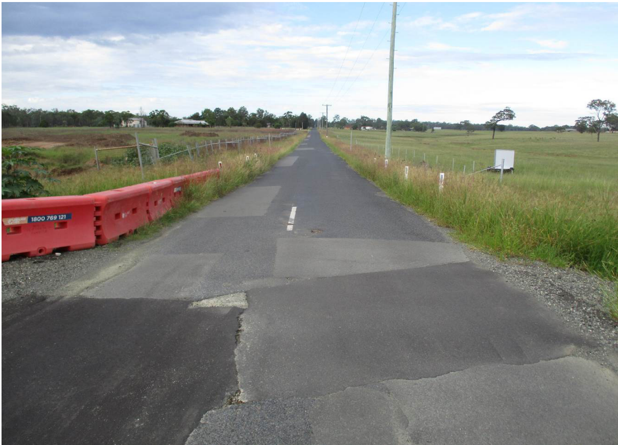
Photograph 5 – Station Lane along site frontage.
