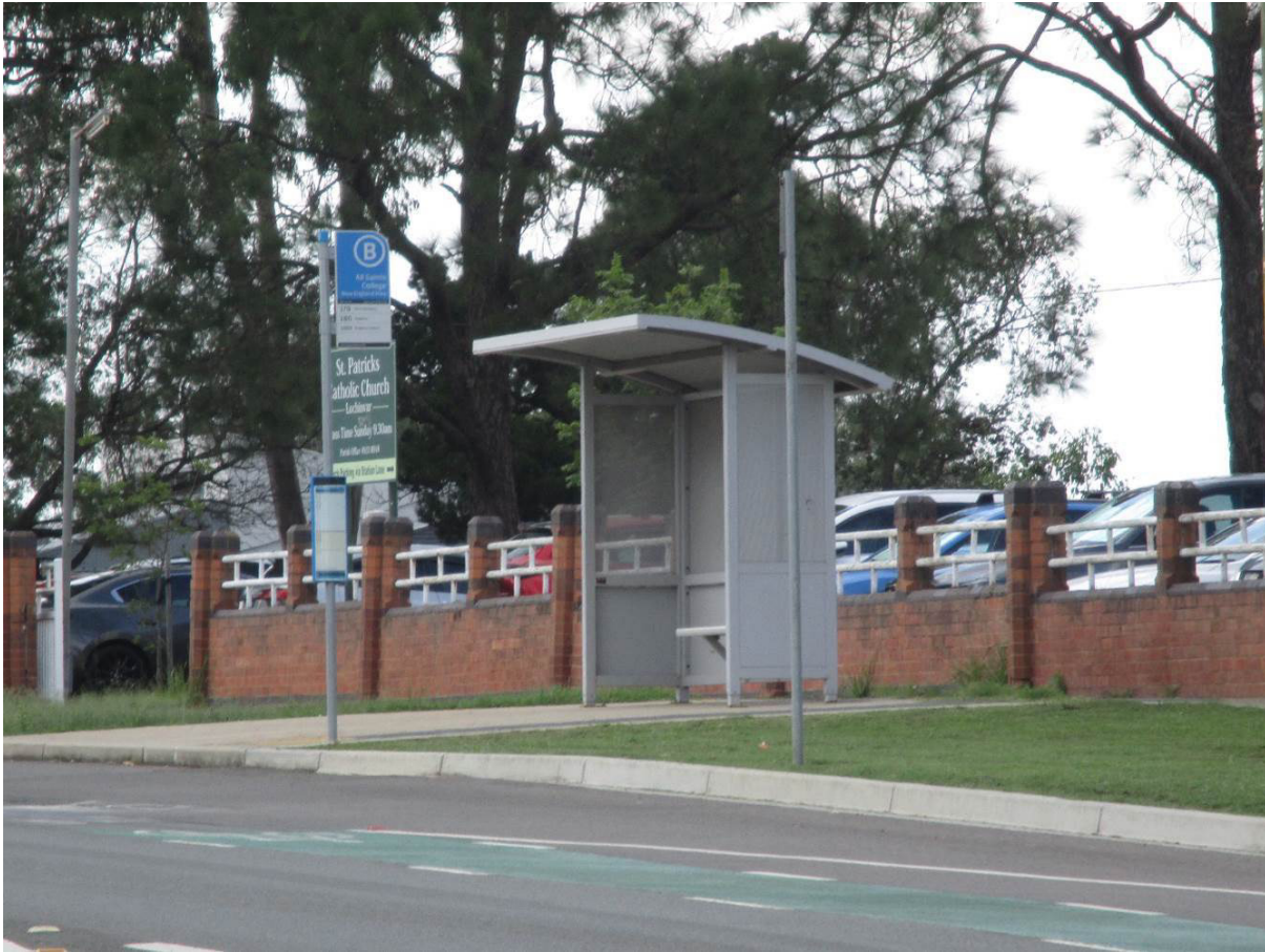
Photograph 8 – Bus Stop on New England Highway near Station Lane.
