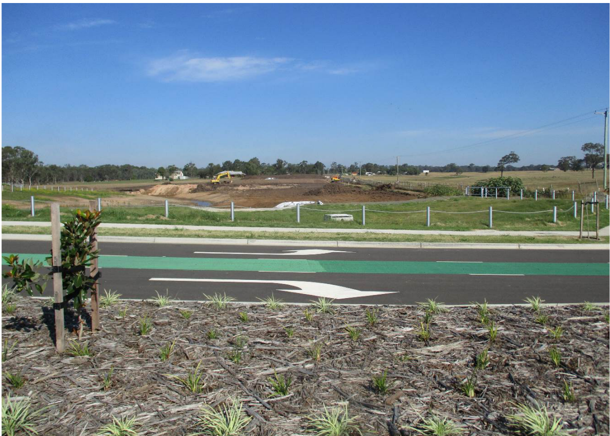
Photograph 2 – Site from Springfield Drive.
