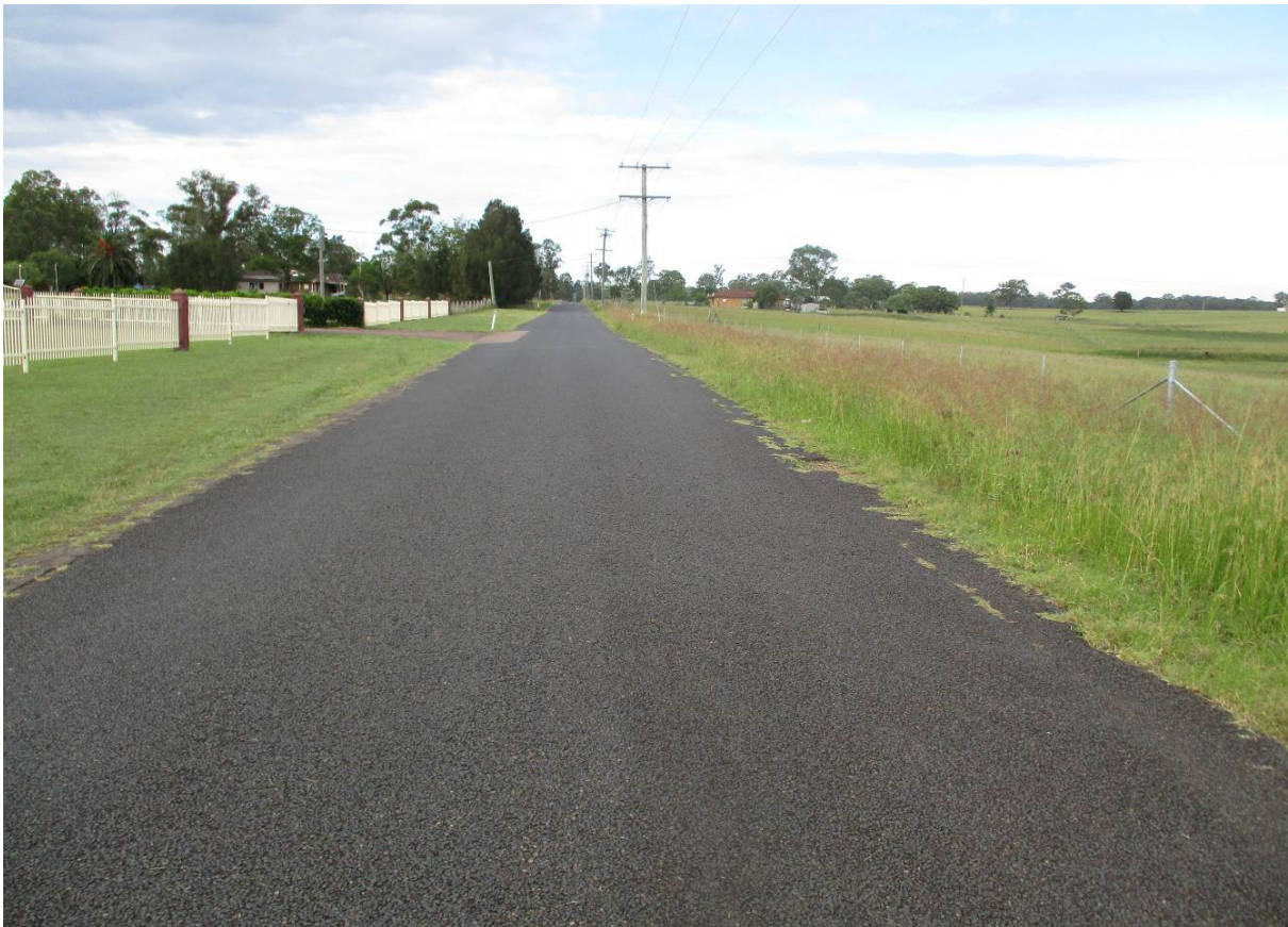
Photograph 4 – Station Lane south of site.
