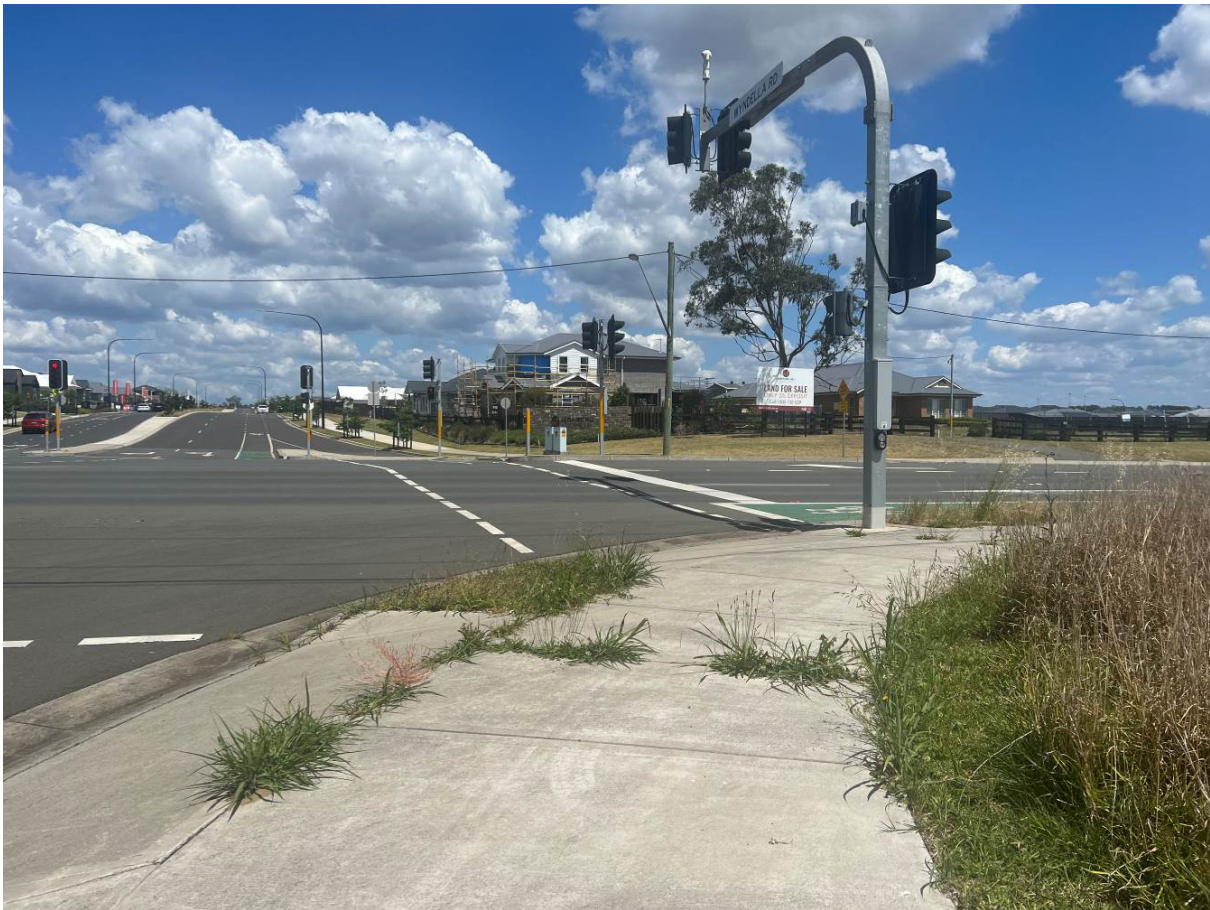
Photograph 6 – Springfield Drive at New England Highway signalised intersection.
