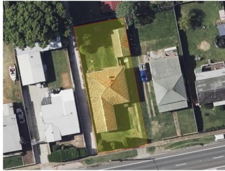
Figure 2 - Existing 236 New England Highway, Site and Context
