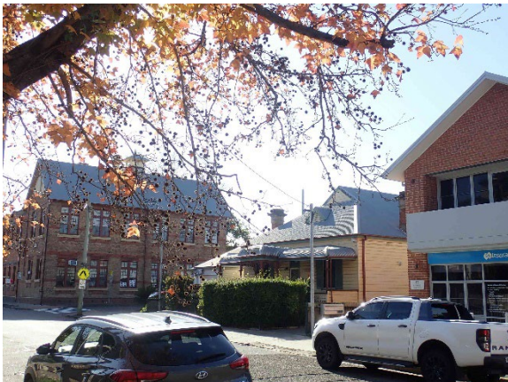
Image 9: Church St 2 storey masonry Source: Placemark 20240704
